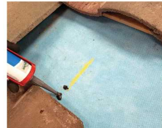
4. Remove hook, clean debris and fill pilot holes with roofing sealant.
