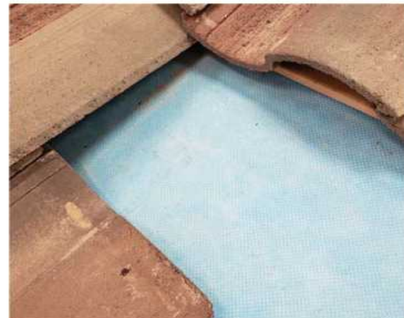
1. Remove tiles around installation area.
