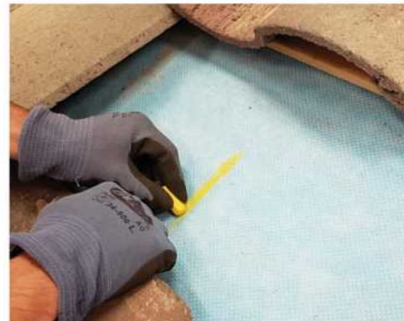
2. Locate and mark rafters.
