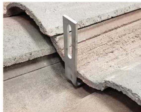
6. Replace tiles, if necessary notch with grinder to ensure proper fit.
