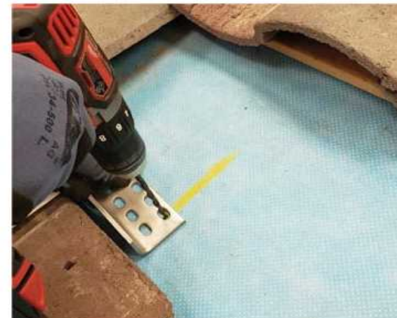
3. Position hook, adjusting arm-base bolt position as needed. Use 3/16" bit to drill 2 pilot holes.
