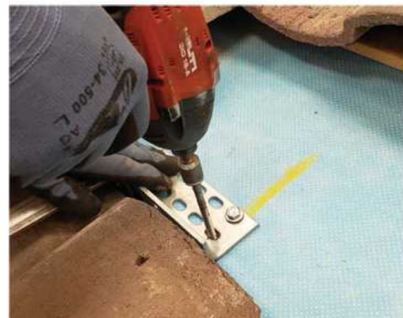
5. Reposition hook, secure with included lag screws.
