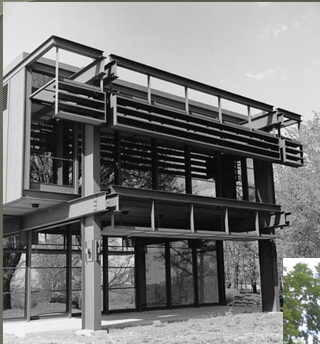
Eero Saarinen's John Deere Headquarters 1964 First use of Cor-Ten in an architectural application
