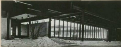
FOREST HOME BRANCH LIBRARY, Milwaukee, Wisconsin Architect: von Grossmann, Burroughs and Van Lanen, Architects, Inc.
