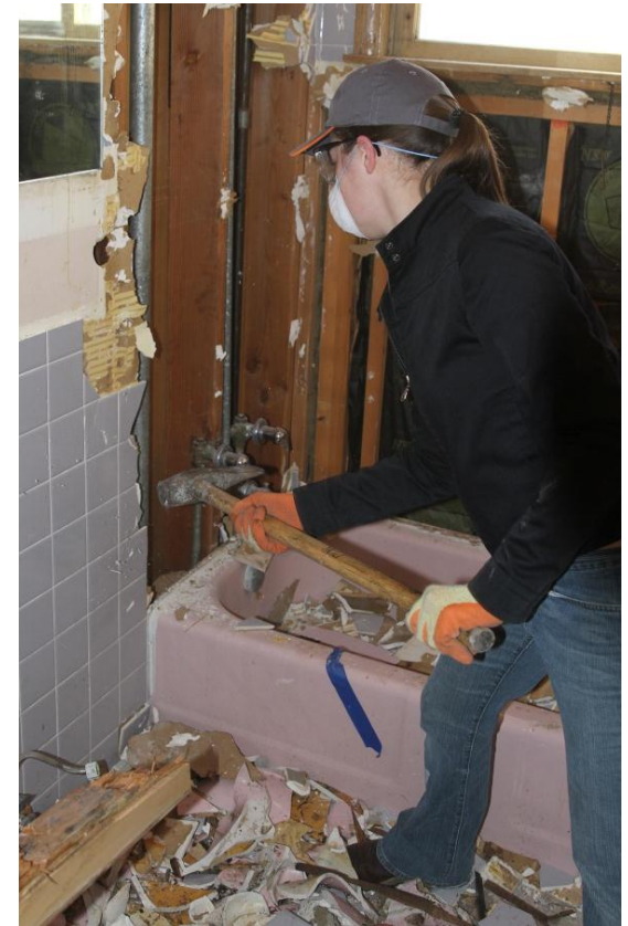
And More Demolition
