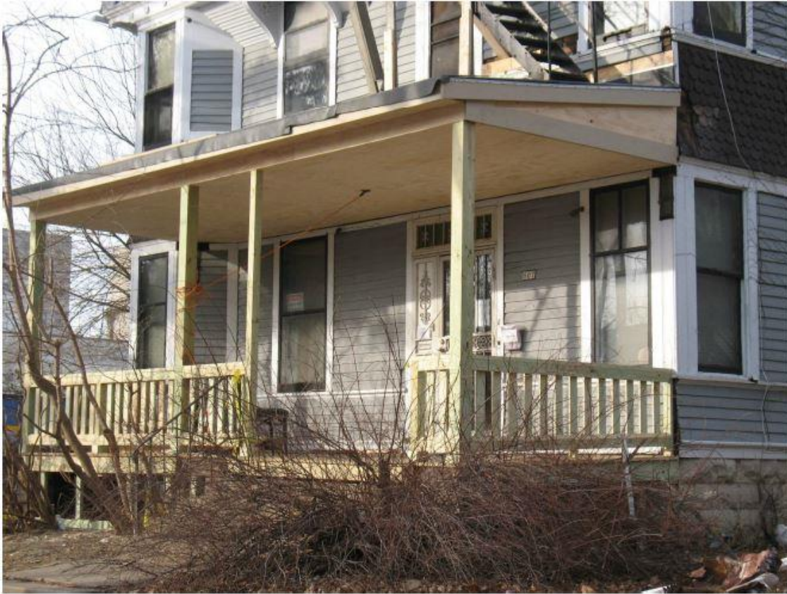
Newly constructed porch 2017
