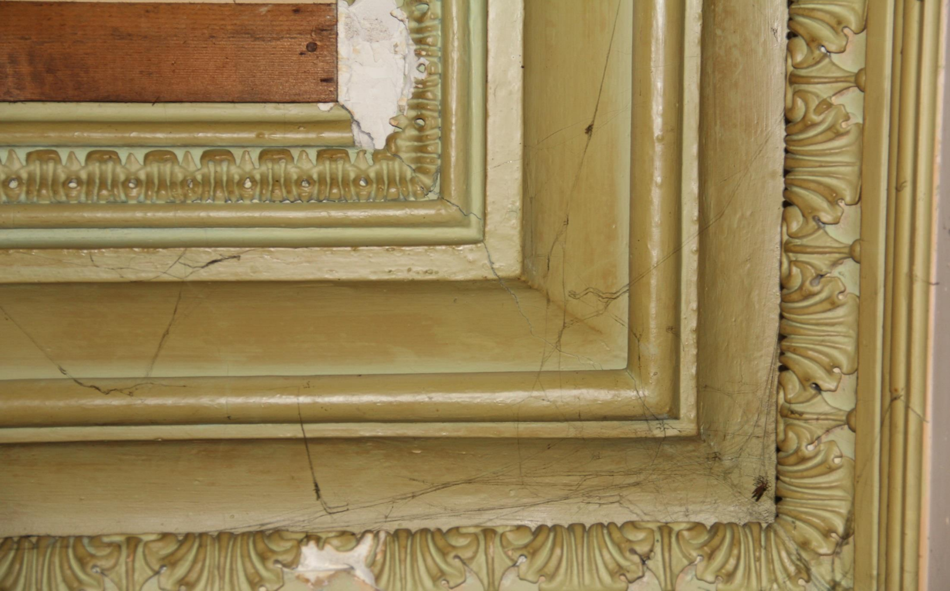
ORNAMENTAL PLASTER CEILING ABOVE DROPPED CEILING
