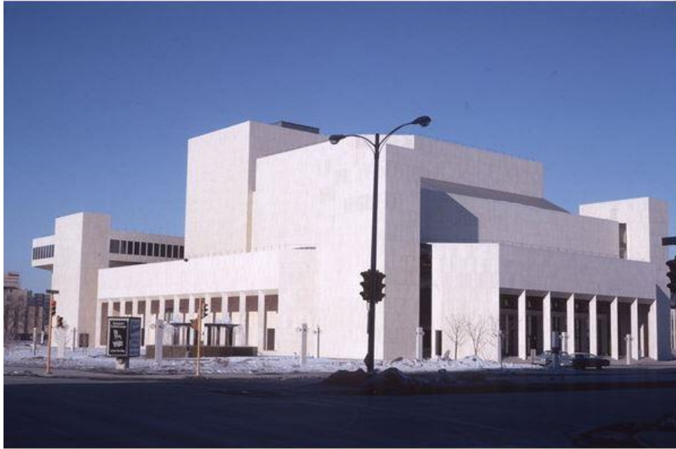
MARCUS CENTER BEFORE REMODELING
