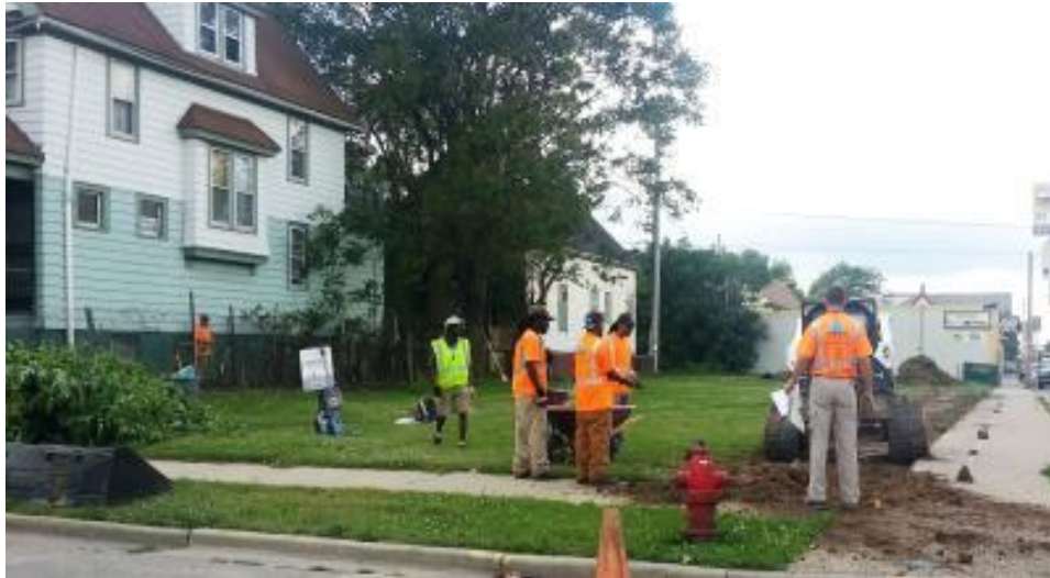
Workers installing green infrastructure
