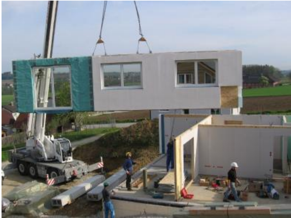
Modular housing being transported to the build site
