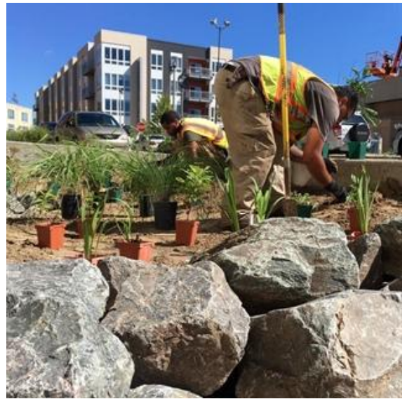
Landscapers installing plants
