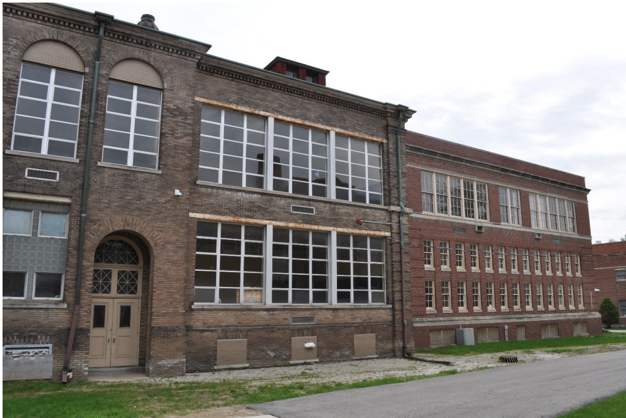
Photo 6 - North elevation of Albrecht Hall and Library
