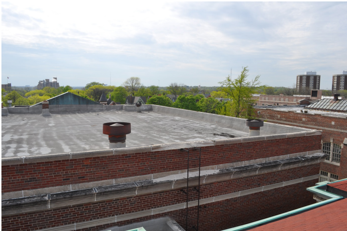
Photo 8 – Library Roof, looking northwest
