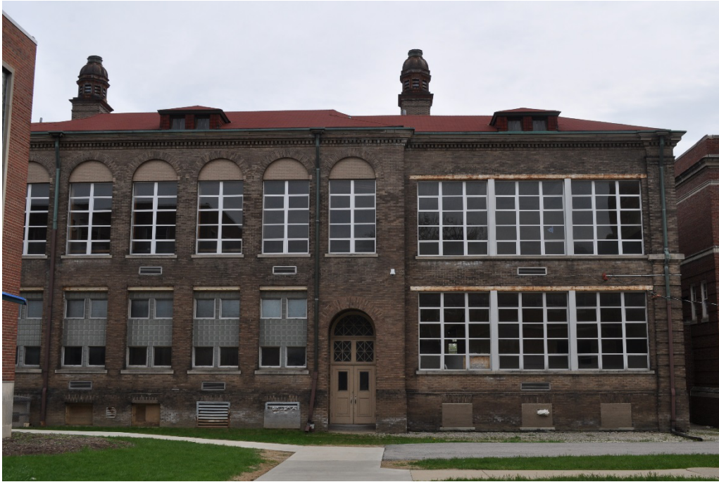
Photo 5 - North elevation of Albrecht Hall
