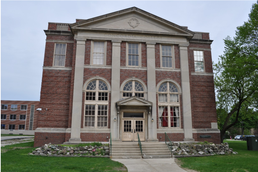
Photo 1 – West elevation of Library
