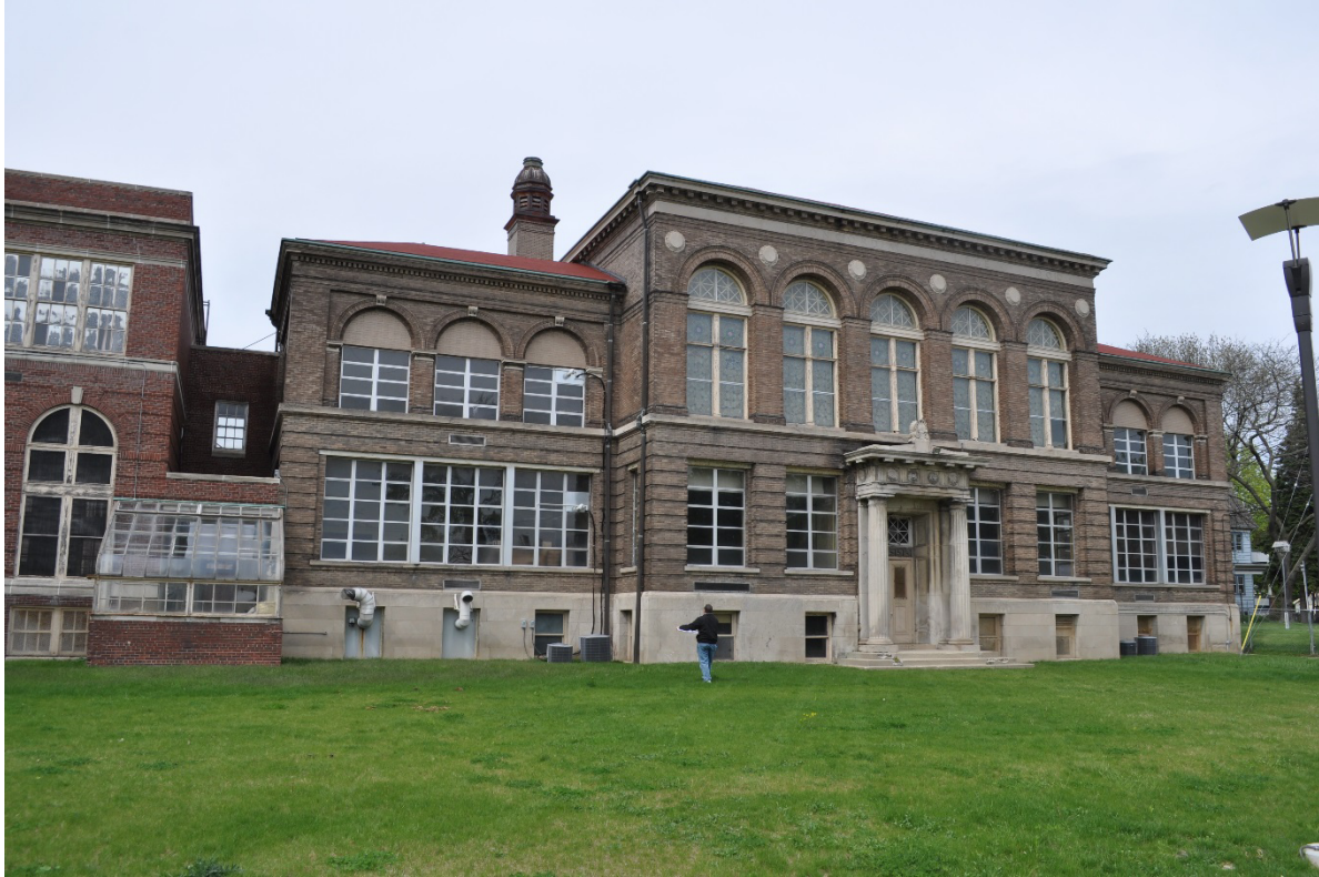
Photo 3 – South elevation of Albrecht Hall
