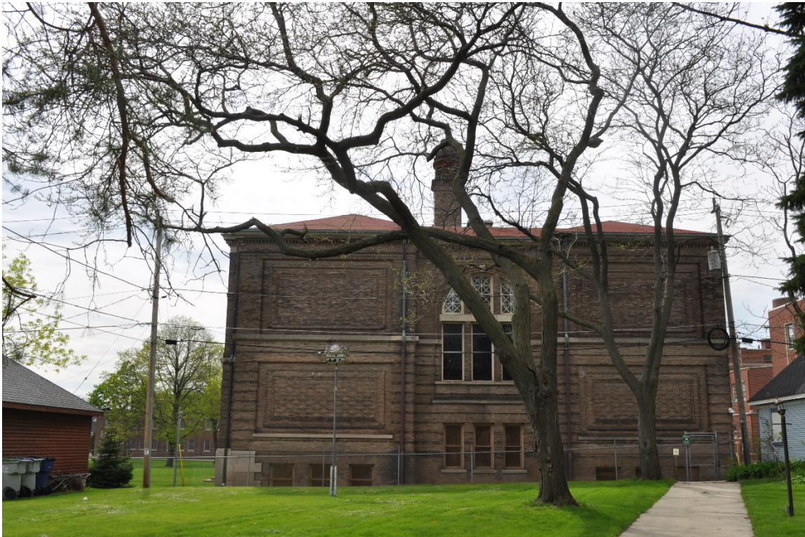
Photo 4 - East elevation of Albrecht Hall
