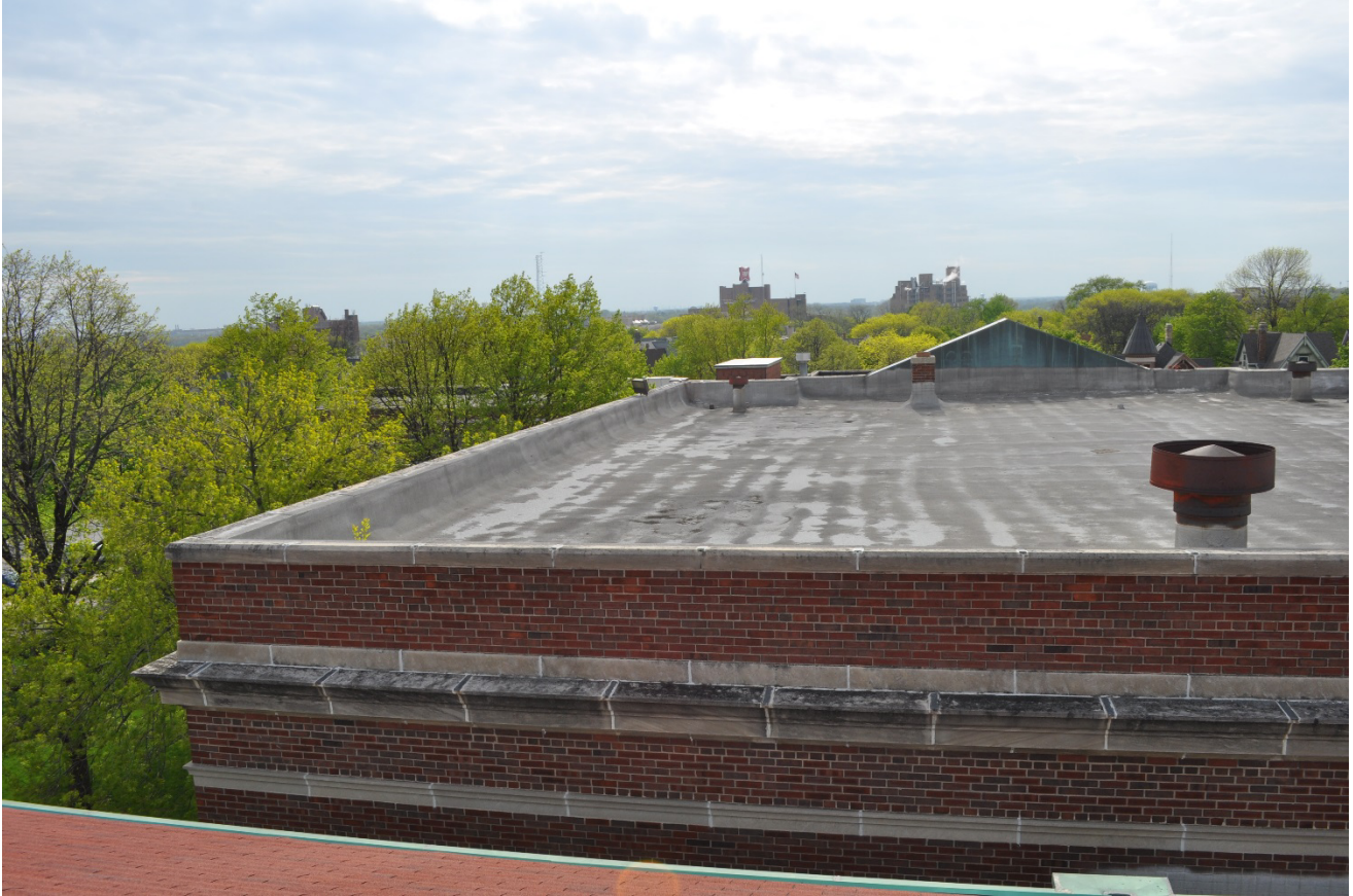
Photo 9 - Library Roof, looking west
