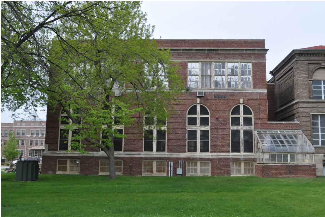
Photo 2 - South elevation of Library
