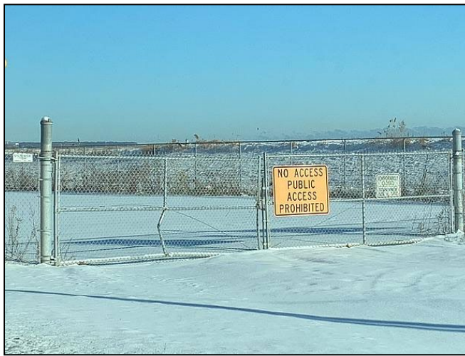
FIGURE C-17.—View of Conflicting Signage Stating no Public Access and Directions for Where Fisherman Should Access Facility.
