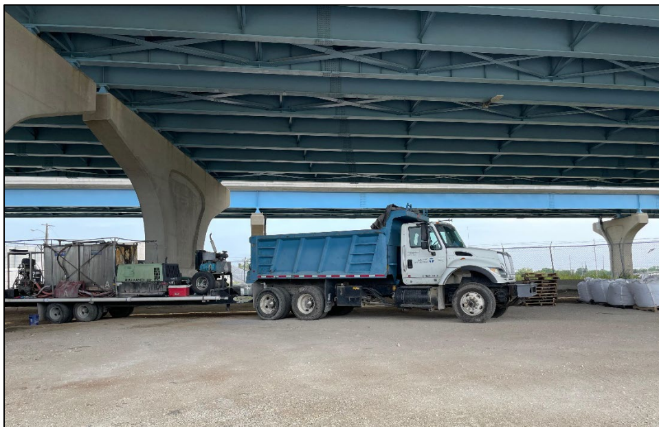
FIGURE 18.—Example of Large Vehicles Parked under I-794 + Hoan Bridge.
