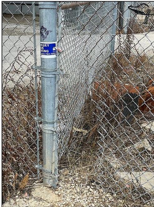
FIGURE C-8.—Example of Perimeter Fence Compromise.
