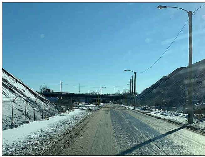
FIGURE C-15.—View Looking South on Carferry Drive at Port Facility Entrance.
