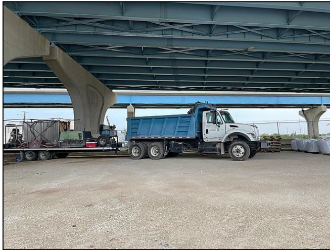
FIGURE C-6.—Example of Large Vehicles Parked under I-794 + Hoan Bridge.
