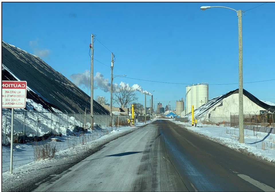
FIGURE 7.—View Looking North on Carferry Drive Showing Open Vehicle Access Gates and Signage Stating to Use Alternate Route when Closed.
