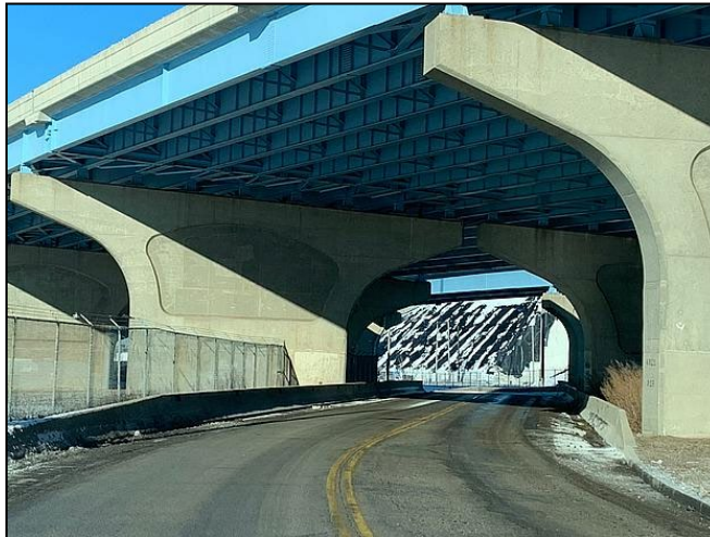
FIGURE C-18.—View of Exposed I-794 Support Structures at Memorial Drive Entrance.
