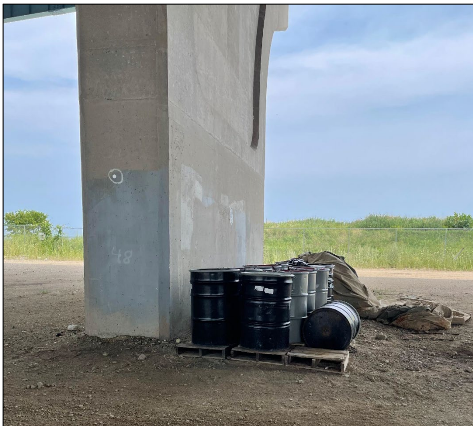
FIGURE 17.—Example of Bulk Liquid Chemicals Stored under I-794 Bridge.
