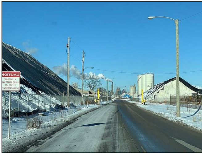
FIGURE C-14.—View Looking N on Carferry Drive Showing Open Vehicle Access Gates and Signage Stating to Use Alternate Route When Closed.
