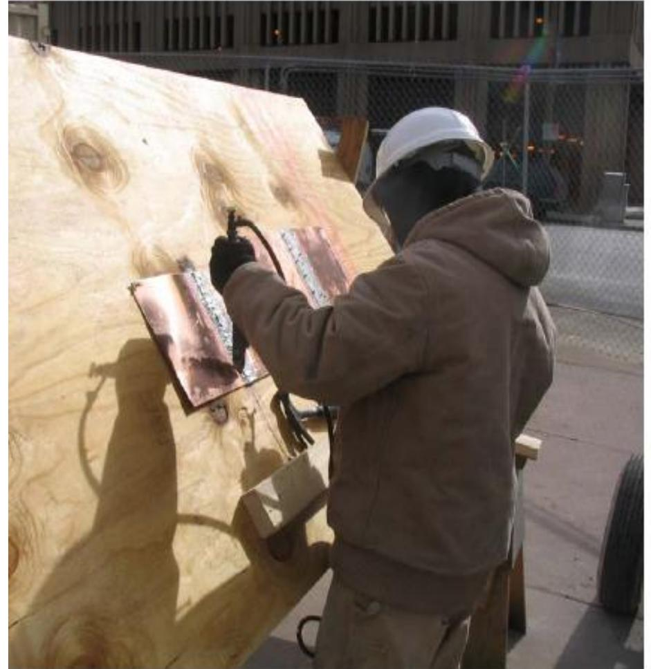
*Mechanic Soldering Test*
