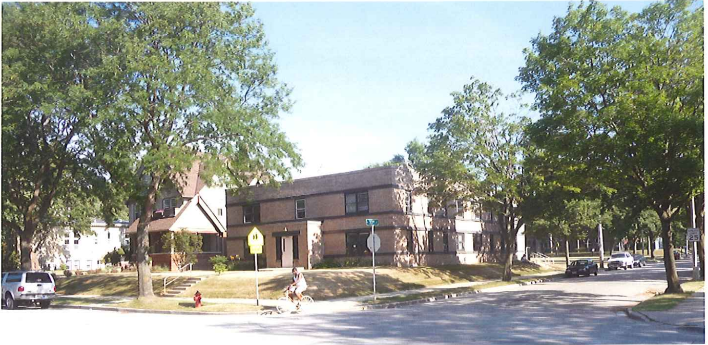
VIEW LOOKING SOUTH EAST FROM WEST HIGHLAND BLVD. AND NORTH 33RD STREET
