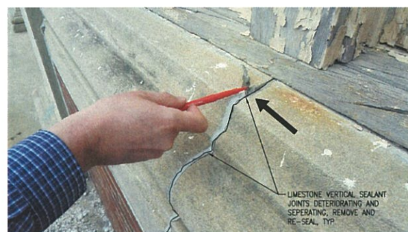
5 VERTICAL SEALANT JOINTS @ LIMESTONE BANDING SCALE: N.T.S.
