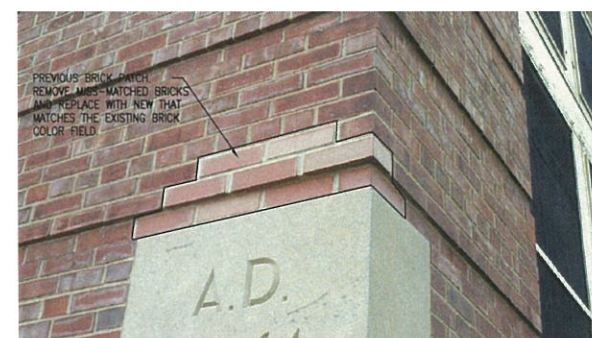
11 NON-MATCHING BRICK PATCH, TYP. SCALE: N.T.S.
