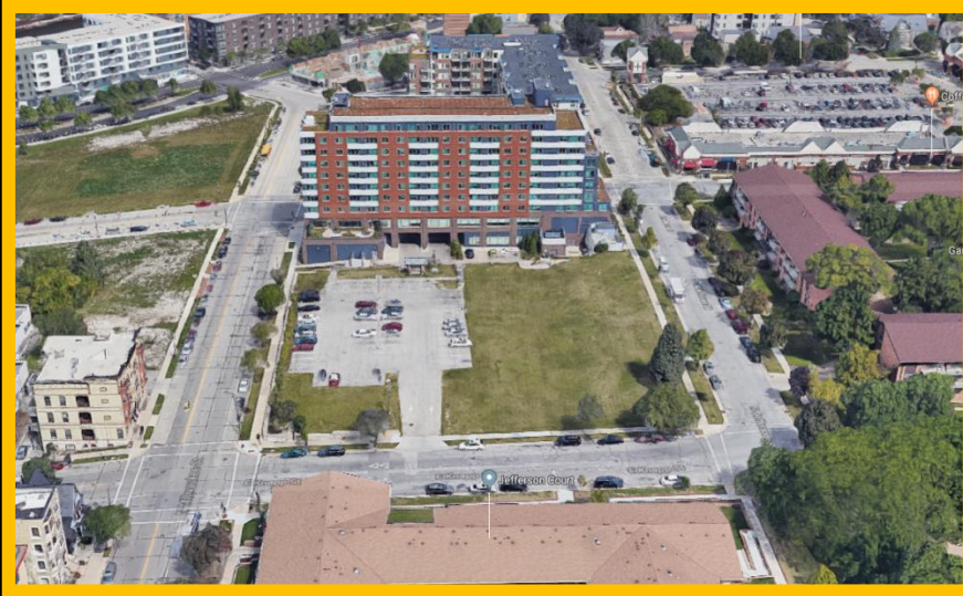
Aerial view looking north
