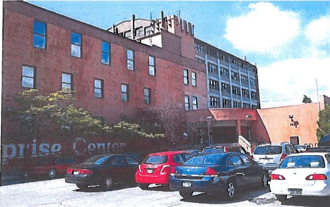
The Welford Sanders Historic Lofts, the proposed redevelopment of a business incubator at 2821 N. 4th St., will be turned into 30,000 square feet of office space and 58 two- or three-bedroom apartments. Credit: Michael Sears
