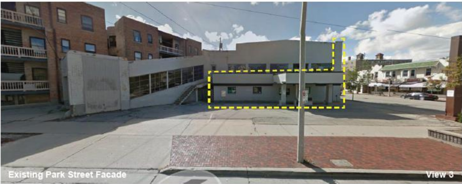
Existing Park Street Facade
