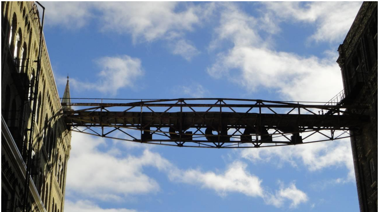
P2 Pabst sign bridge (looking east)
