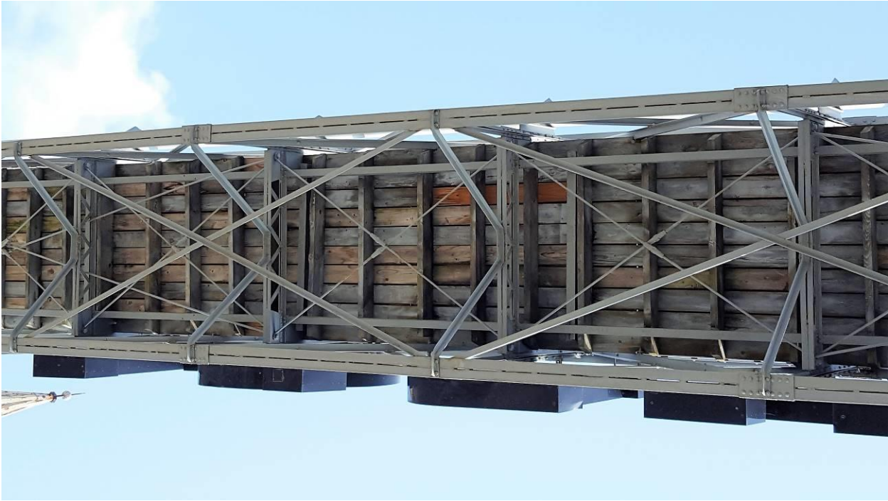
P3 Pabst sign bridge (bottom view).
