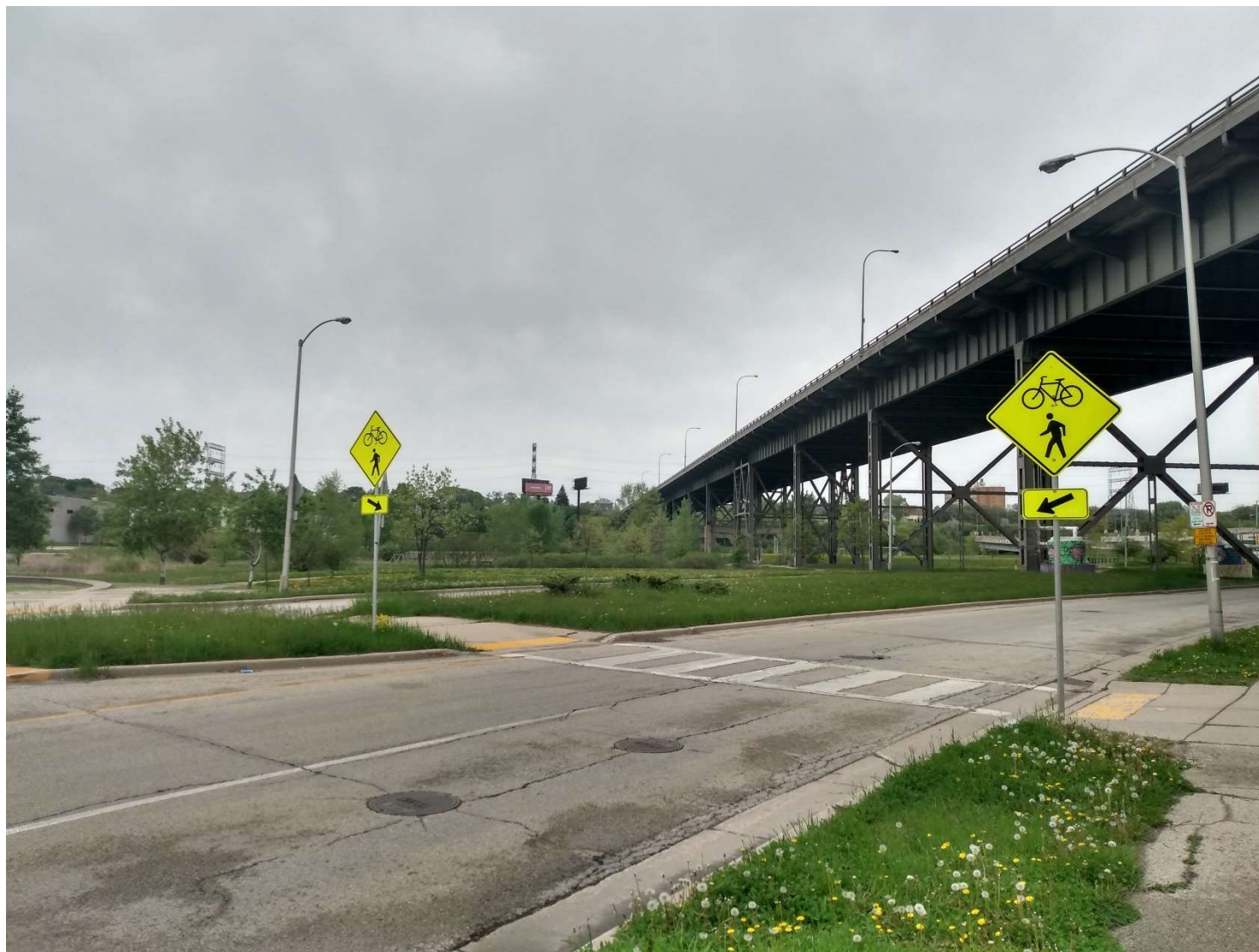
Picture D: The HAST crossing in the Menomonee Valley, looking northwest. Here, the signs alert drivers to both pedestrians and cyclists.
