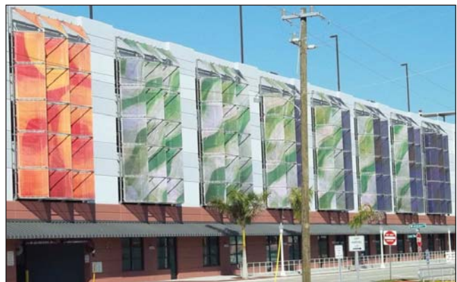
Figure 35. Artistic panels used to enliven traditional parking garage facade in Fort Myers, FL.
