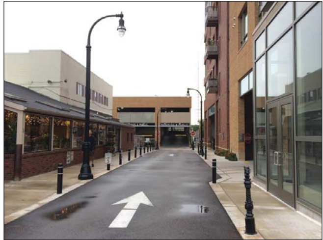
Figure 34. The Parking structure at LightHorse 4041 Apartments in Shorewood, WI is available to both residents and retail customers.
