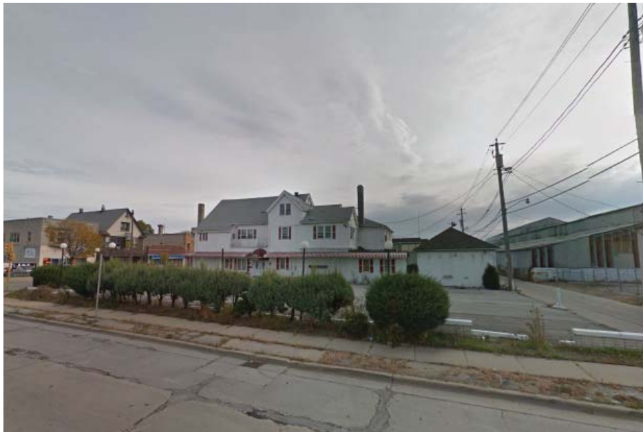
View West from N. 37th Street
