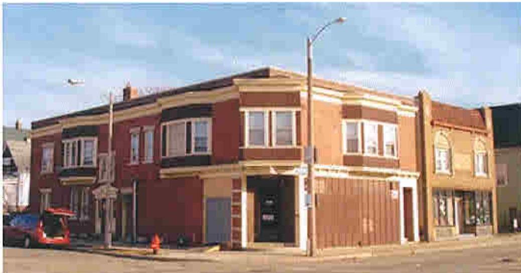
This building (3832 West Lisbon Avenue) is located just east of the Development Site.
