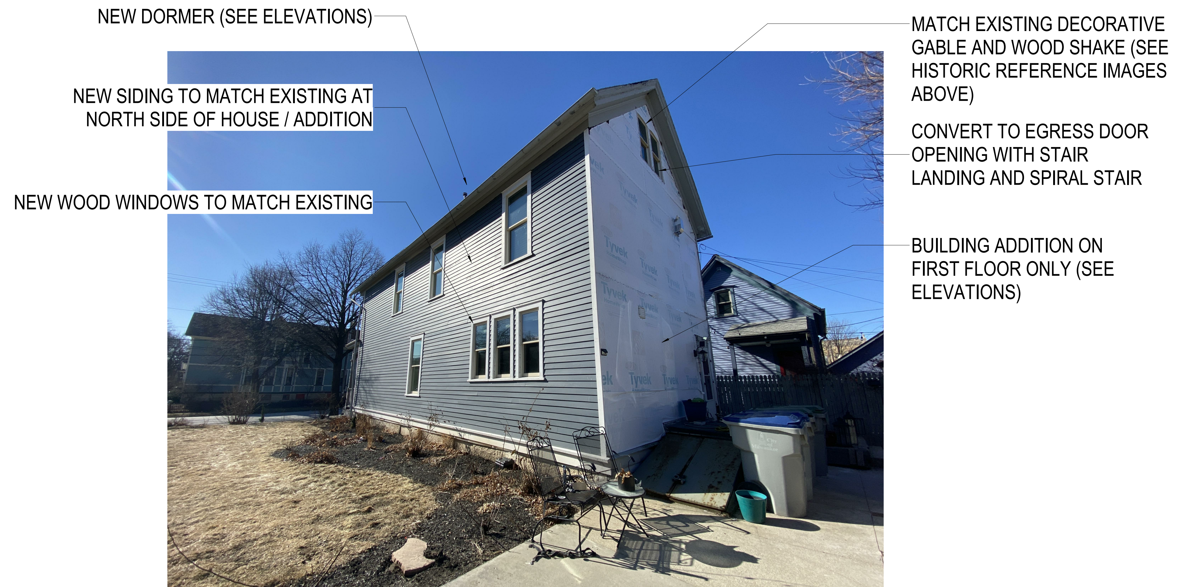
1 PHOTO - NE CORNER OF HOUSE 1 1/2" = 1'-0"
