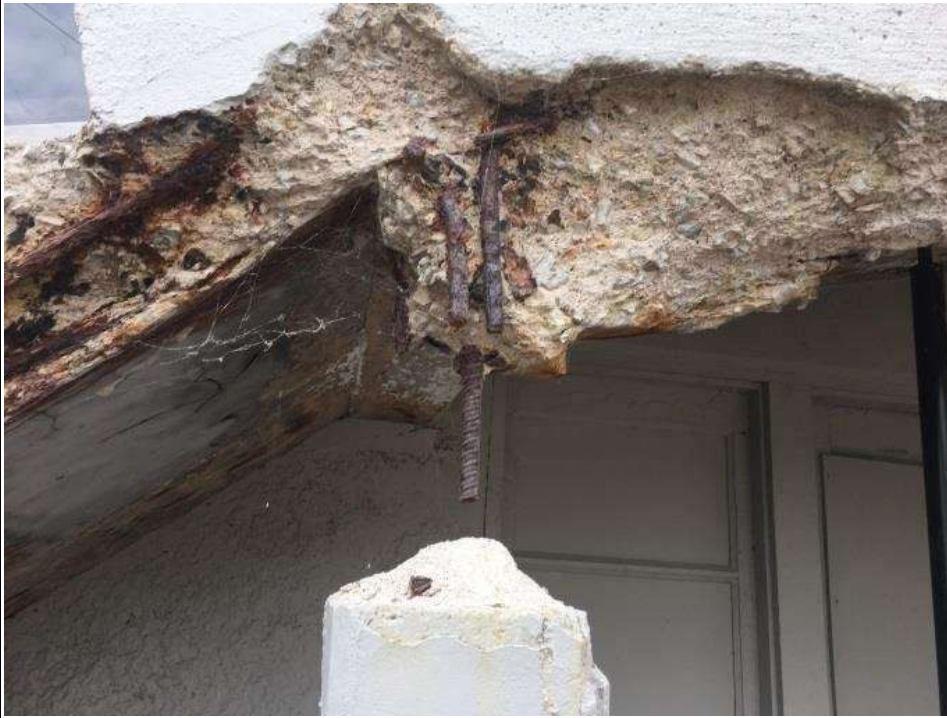
Details of major deterioration showing temporary shoring posts (black).
