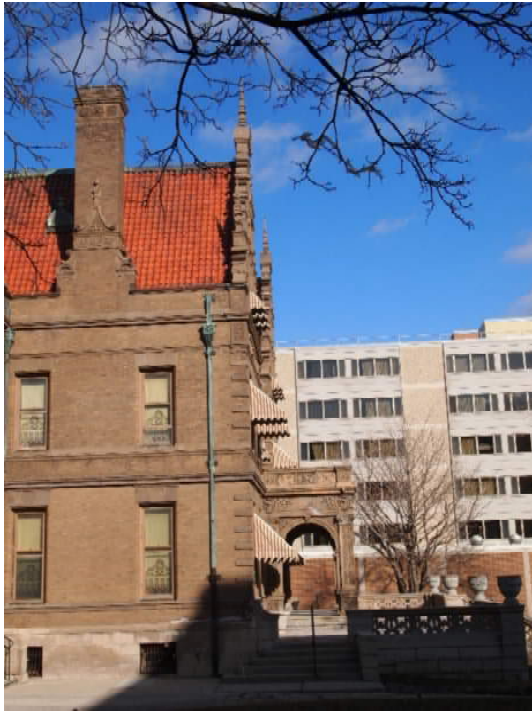
West Elevation Chimney
