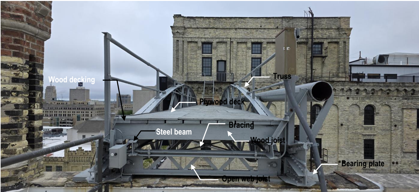
P4 Pabst sign bridge decking (looking south).
