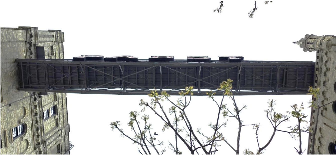
P3 Pabst sign bridge (bottom view).
