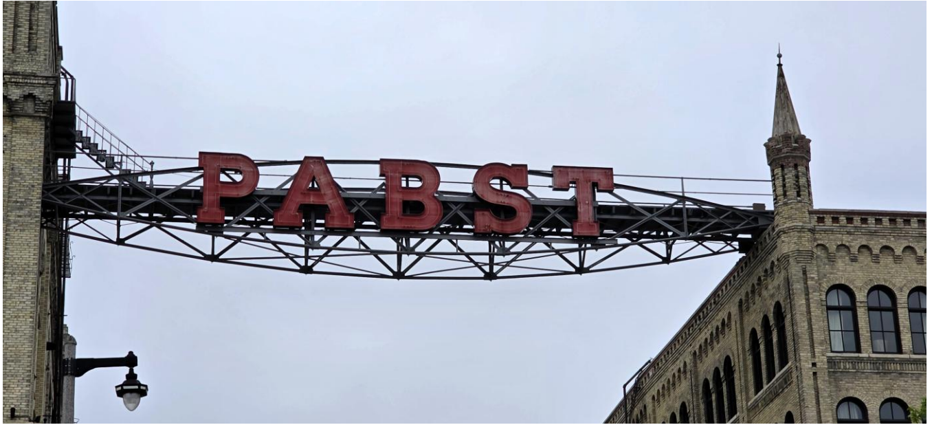
P1 Pabst sign bridge (looking west)
