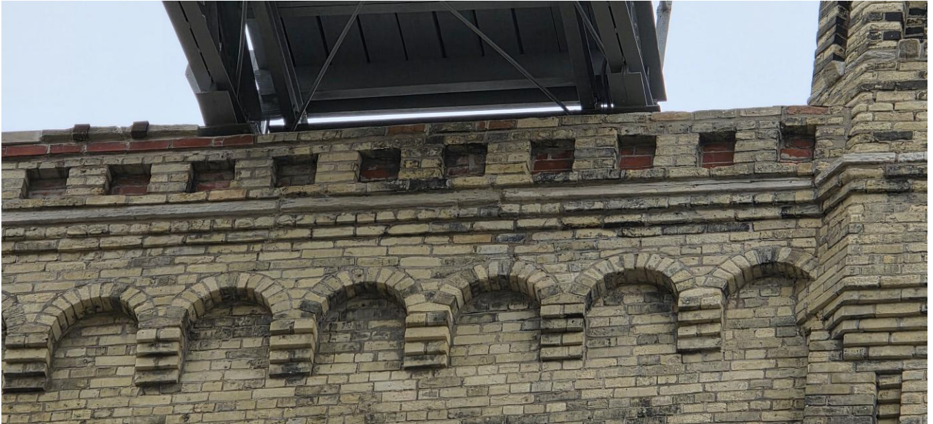
P7 Pabst sign bridge north support end.
