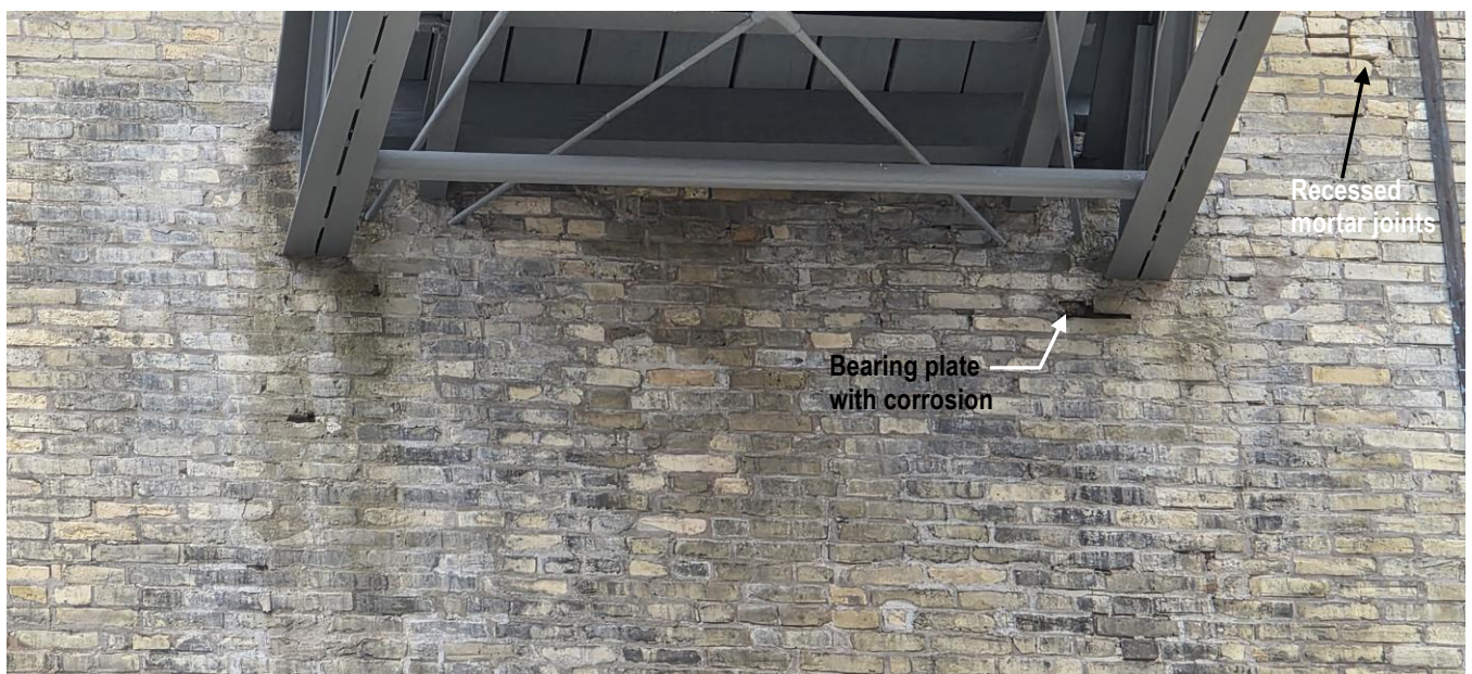
P6 Pabst sign bridge south support end
