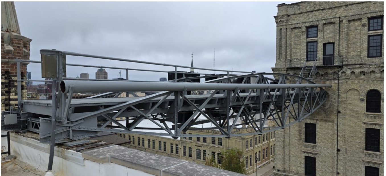
P2 Pabst sign bridge (looking east)
