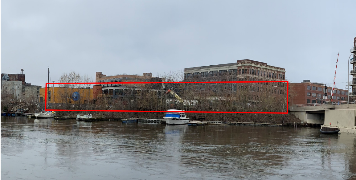
View South Across River
