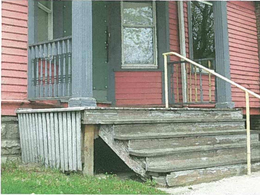
3. Front Porch (East Elevation) skirt and stairs
