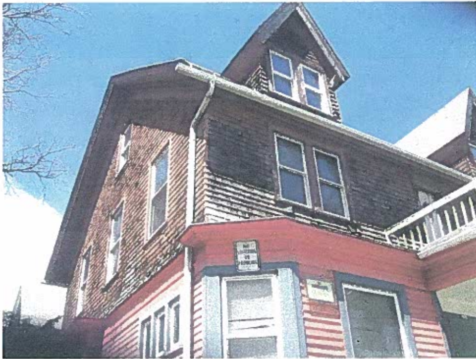
1. Front (East Elevation) w/ shingled upper level, two dormers, porch railing & K Style gutters
