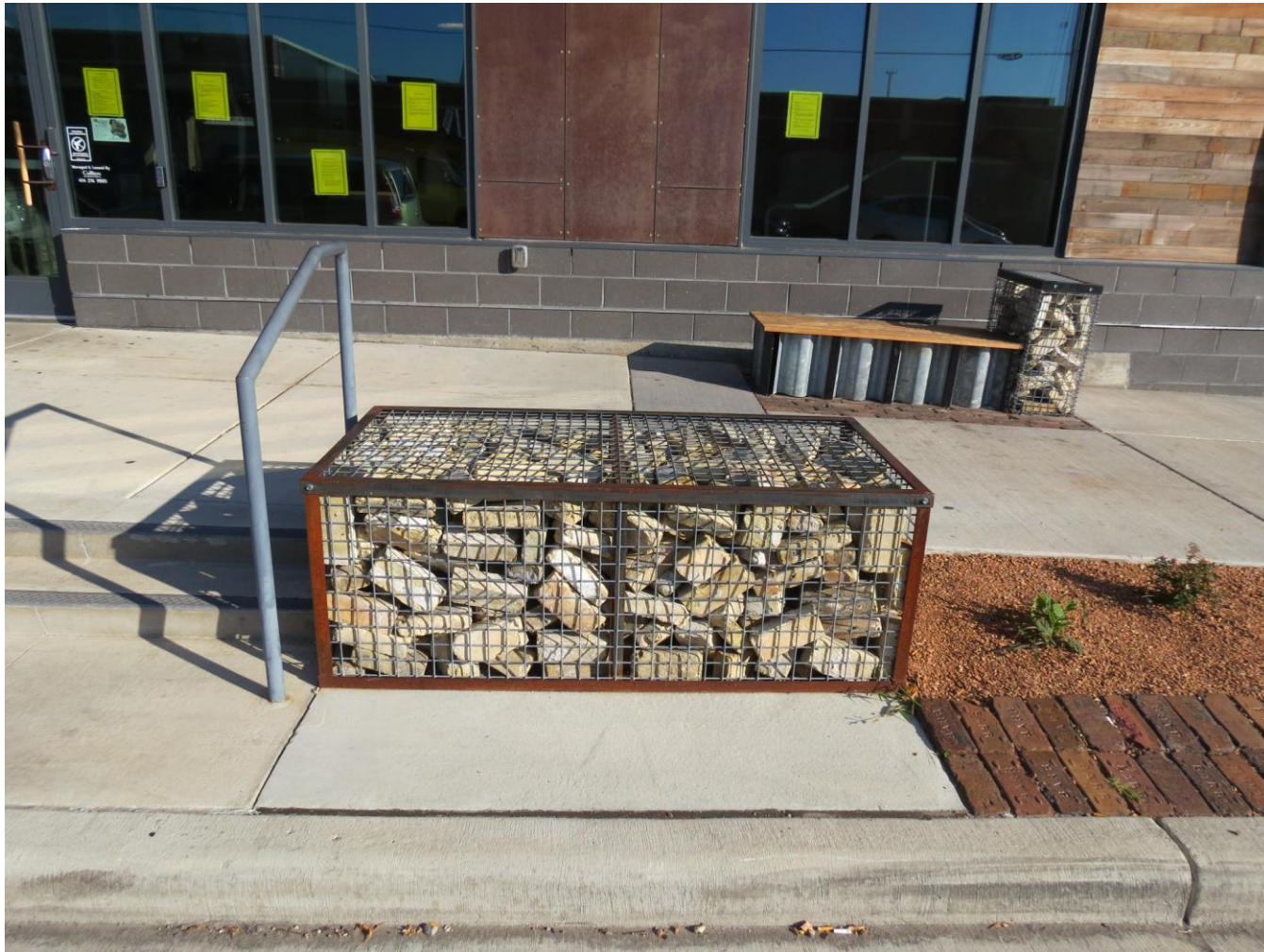
CCF 111744 Close up of a gabion.
