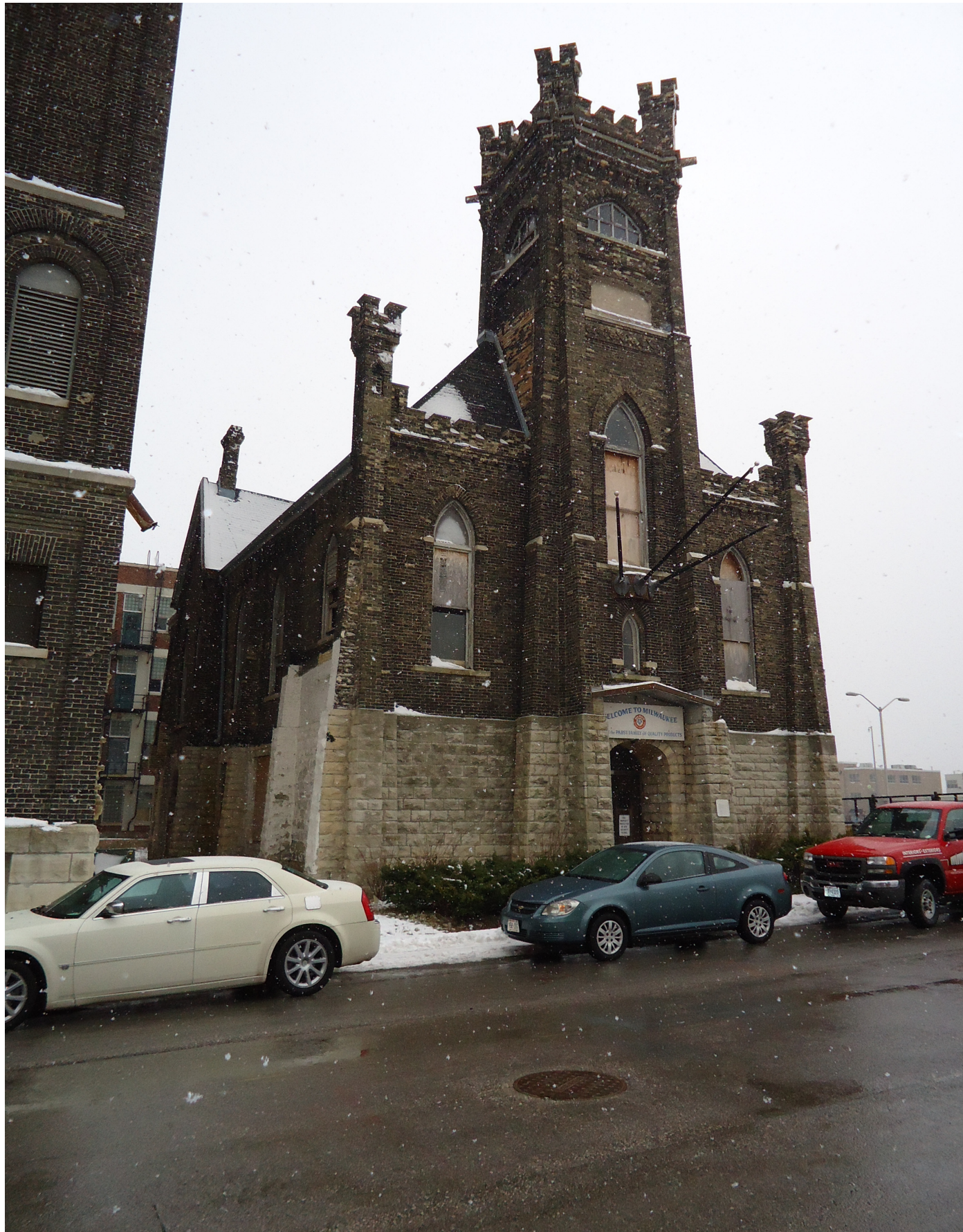
EXISTING FIRST GERMAN METHODIST CHURCH TO THE SOUTH
