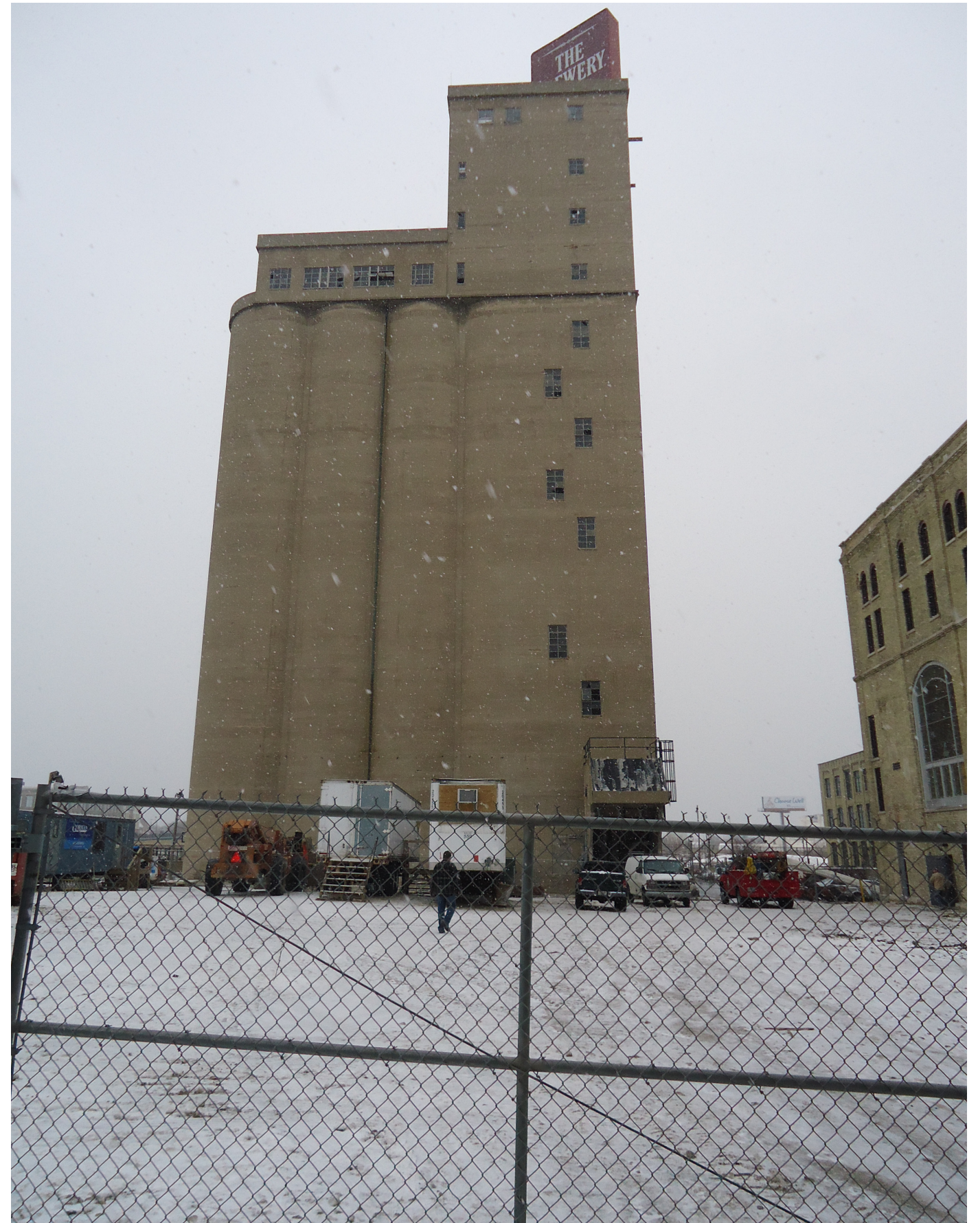
EXISTING CONCRETE GRAIN SILOS TO THE NORTH
