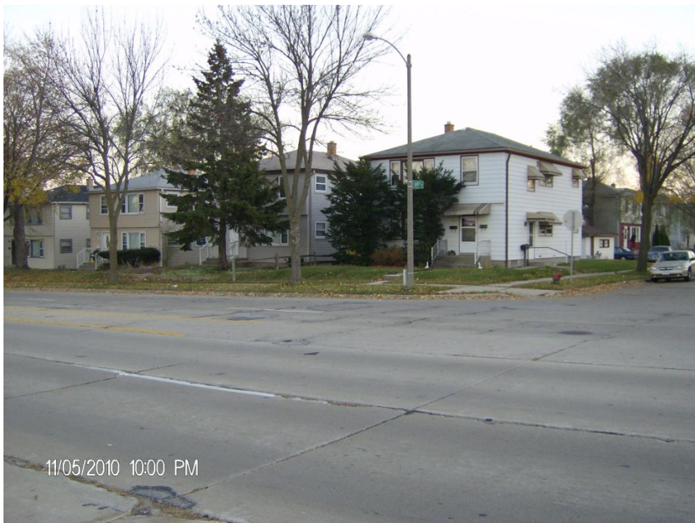
W. Florist Avenue, looking southeast from the DPD site
