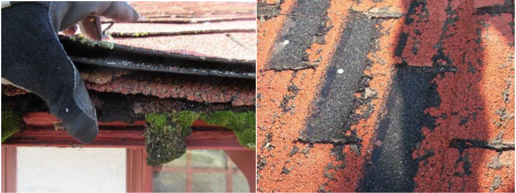
Typical existing conditions as of 3/25/2016.
