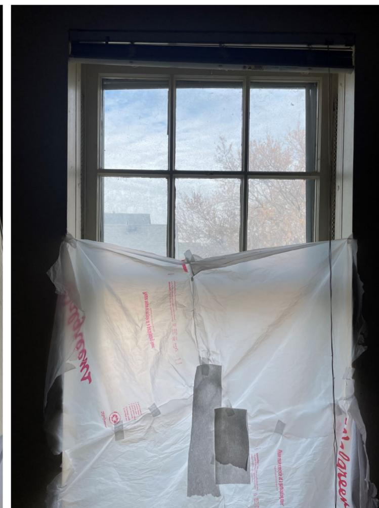
Storm windows are outfitted on all windows to temper the heat transfer with the single-pane glass windows. Despite this, the draft through the windows is extremely uncomfortable for the senior aged residents. The property manager uses painter's tape to seal all the window joints. This particular tenant used plastic bags to create an additional weather barrier.
