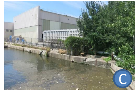
Milwaukee Recycling Facility Building and truck traffic / storage <25' from water edge
