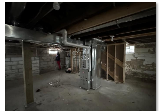
4369 N 26 th Street - Basement
