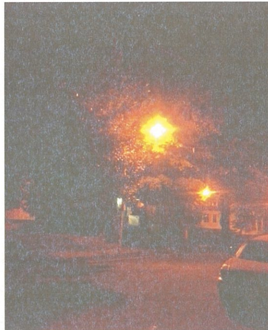
Lights were obstructed by overgrown trees.
