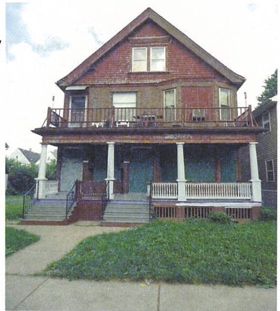
This is one of four boarded up properties on the block.
