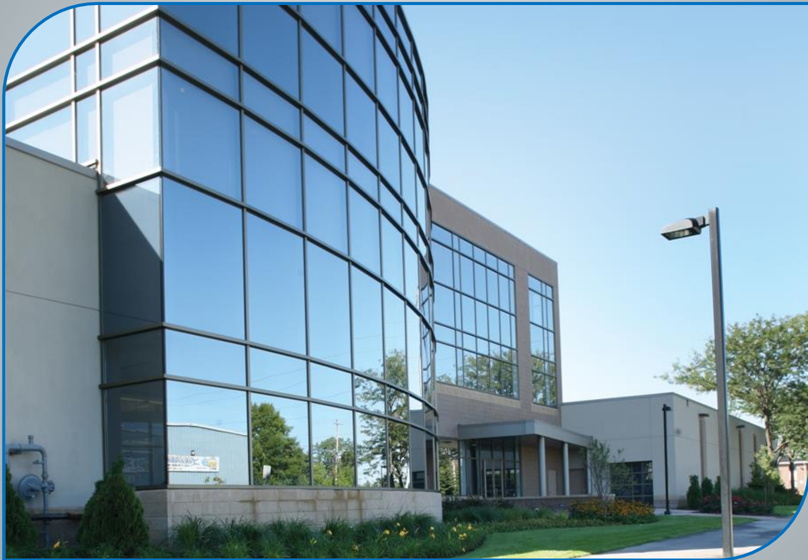
3-story Building 1.5 on Direct Supply's global headquarters in Milwaukee, Wisconsin
