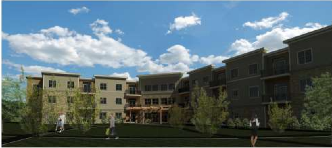
APPROXIMATE VIEW FROM INNER COURTYARD
