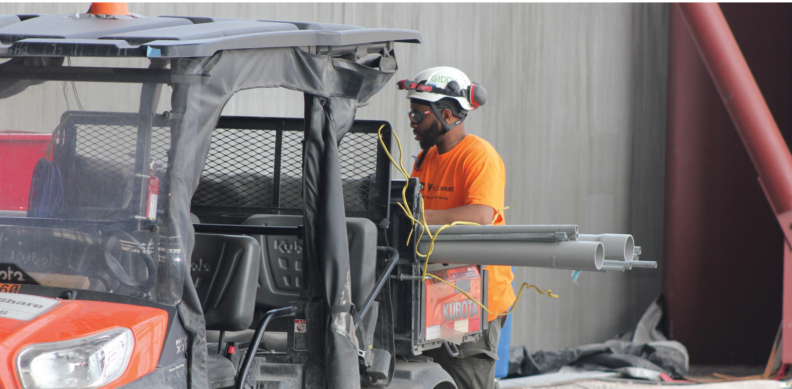
Pipefitter preparing to transport materials to new work station.
