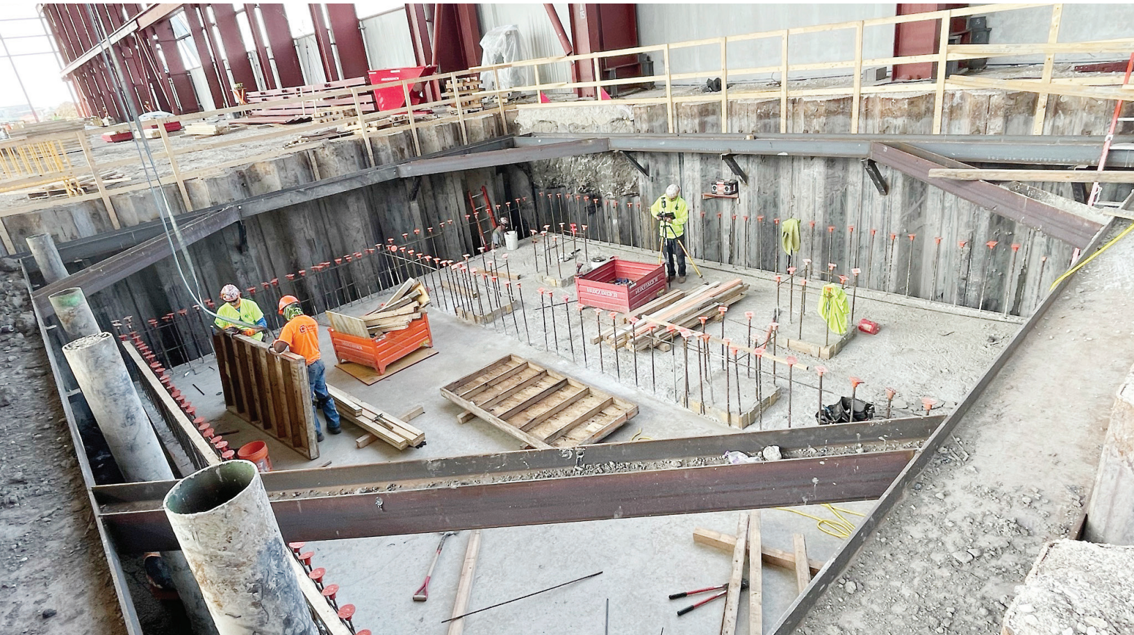
Trade workers making progress.
