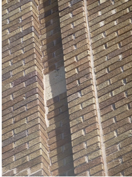
Photo 3 - 5.18.15: Masonry articulation on southeast corner of main building
