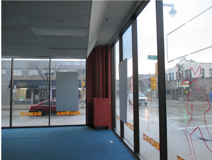
Photo 17 - 12.23.14: Interior view of storefront windows, looking southeast
