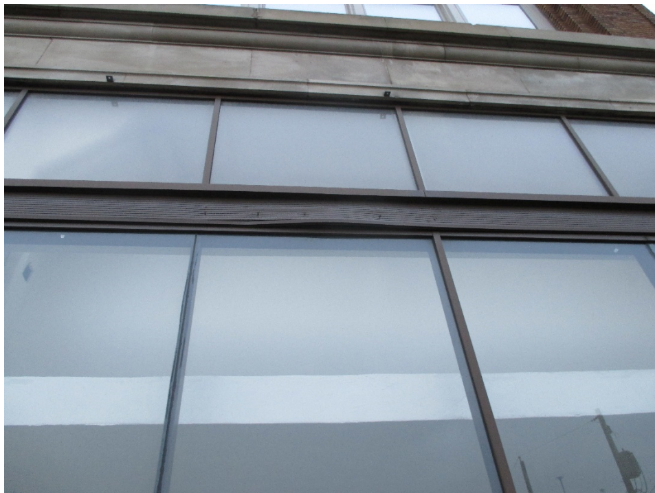
Photo 16 - 12.23.14: Storefront windows on east elevation of building
