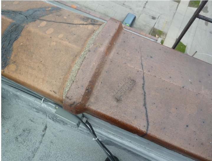
Photo 9 - 5.12.15: Ceramic coping on top of main building roof
