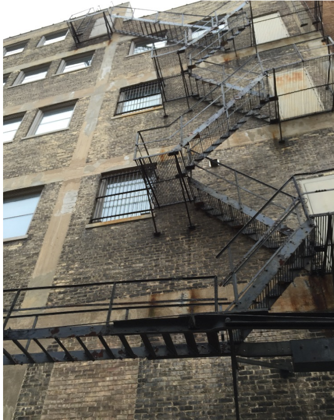
Photo 13 - 5.12.15: Fire escape stairs located at west elevation of main building
