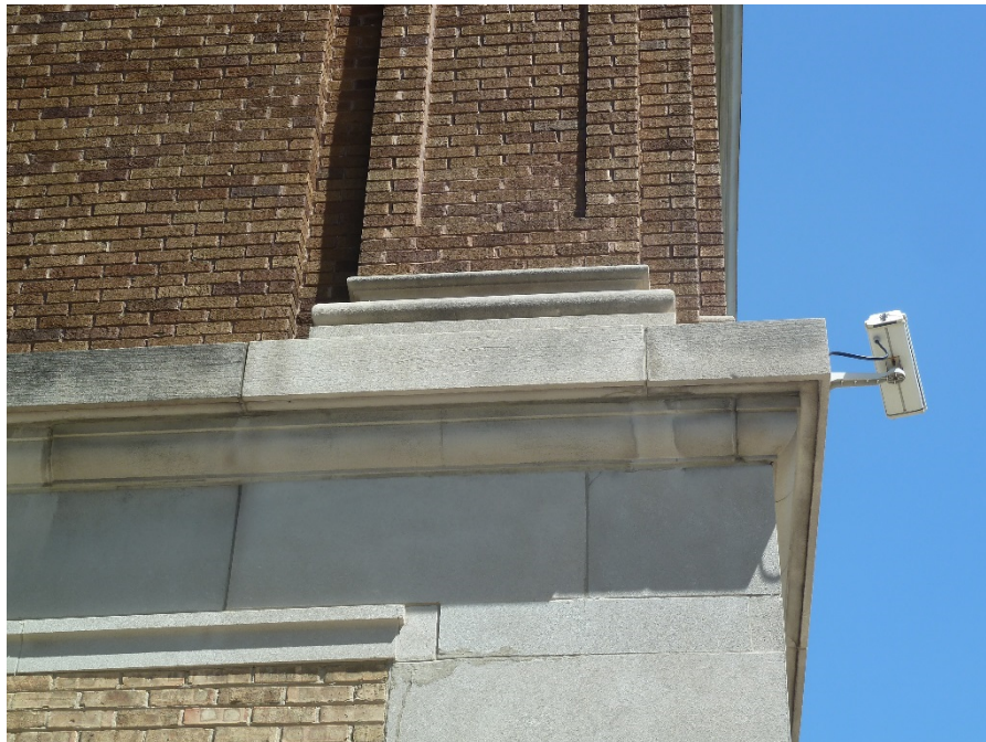
Photo 4 - 5.18.15: Existing limestone sill on southeast corner
