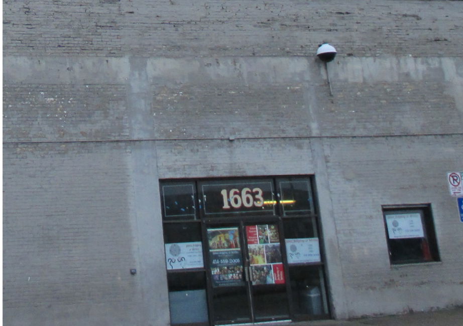
Photo 21 - 12.23.14: North elevation entry of storage building
