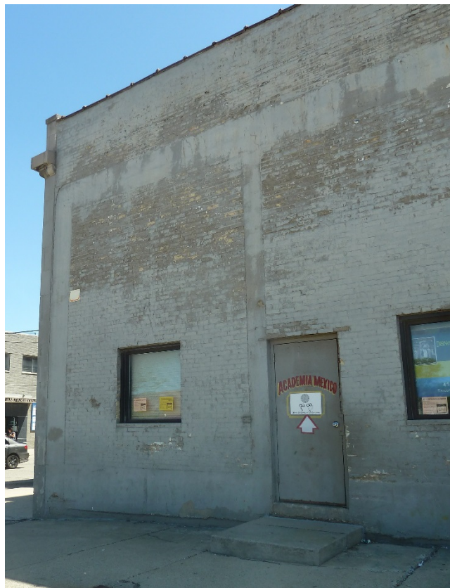
Photo 22 - 5.18.15: Side entrance on north elevation of storage building
