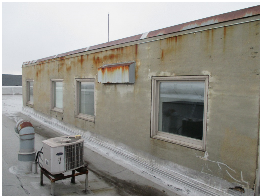
Photo 8 - 12.23.14: 5 th floor, east façade
