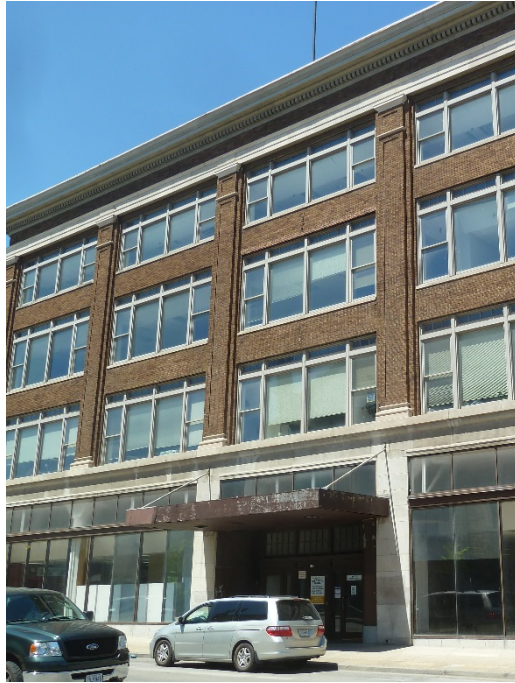
Photo 19 - 5.18.15: Main entrance on south elevation, canopy to remain during construction
