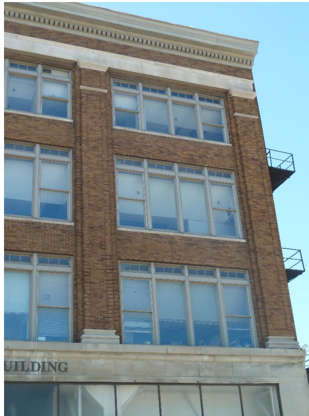
Photo 15 - 5.18.15: Window details on east façade of main building
