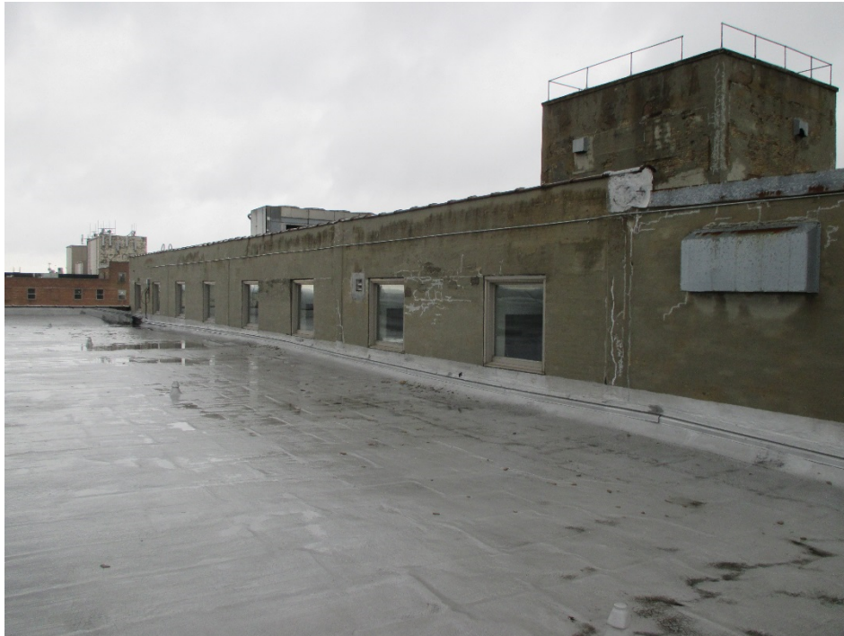
Photo 7 - 12.23.14: Main building roof looking northwest toward 5 th floor
