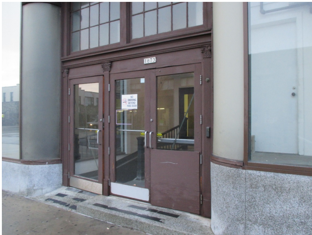
Photo 18 -12.23.14: Building entry on east elevation
