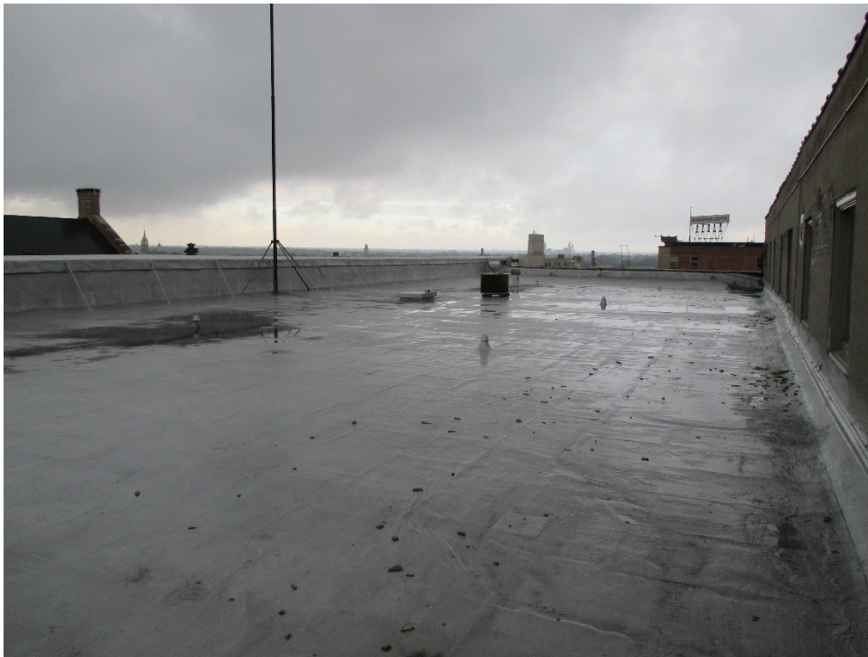
Photo 6 - 12.23.14: Main building roof looking southwest
