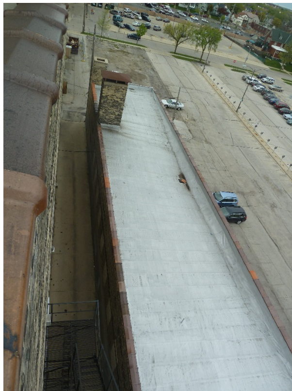
Photo 12 - 5.12.15: View of north building roof, looking northwest
