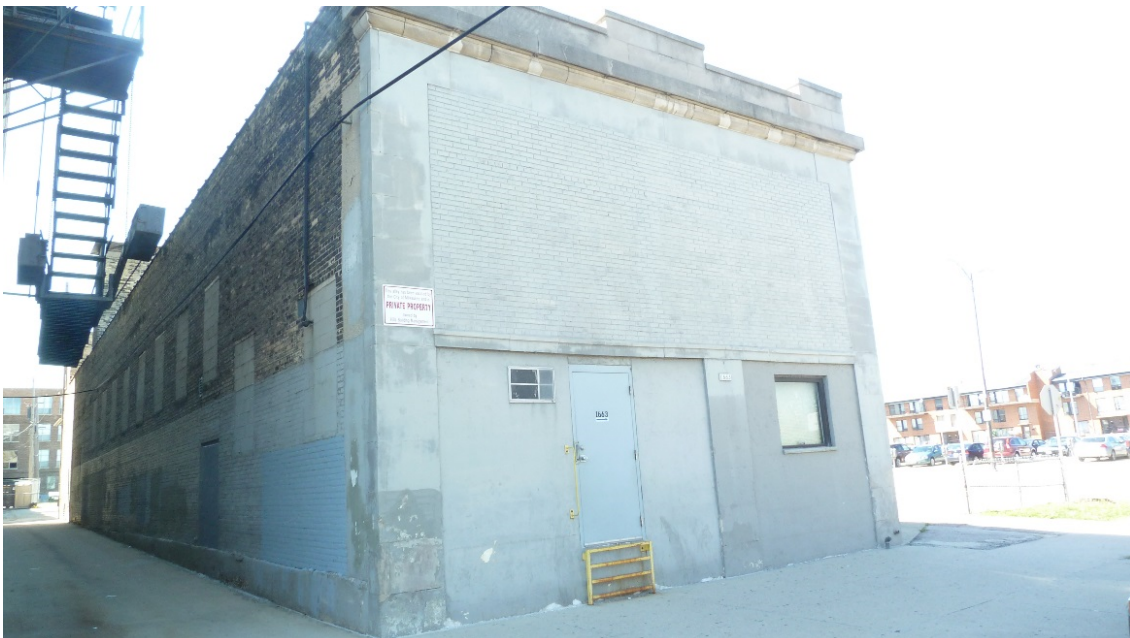
Photo 2 - 12.23.14: Storage Building, east façade, looking northwest
