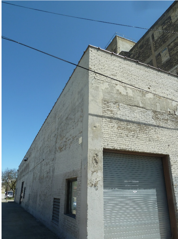
Photo 23 - 5.18.15: Overhead door on west elevation of storage building
