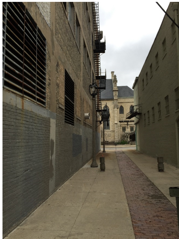
Photo 26 - 5.12.15: West façade, main building, and public walkway/ vacated alley
