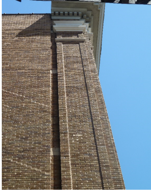
Photo 5 - 5.18.15: Existing limestone cornice on southwest corner
