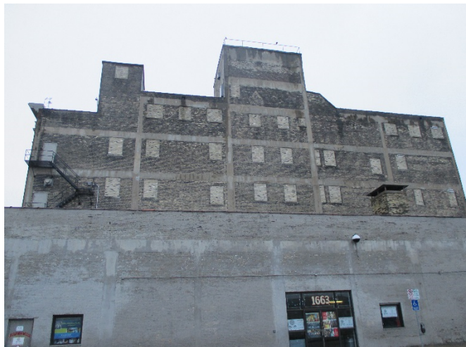
Photo 20 - 12.23.14: North facades, storage building and main building
