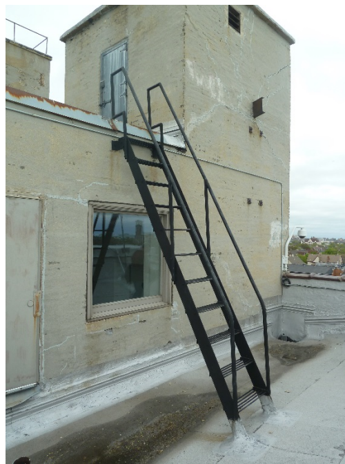
Photo 10 - 5.12.15: Stairway to 5 th floor roof on north side of main building
