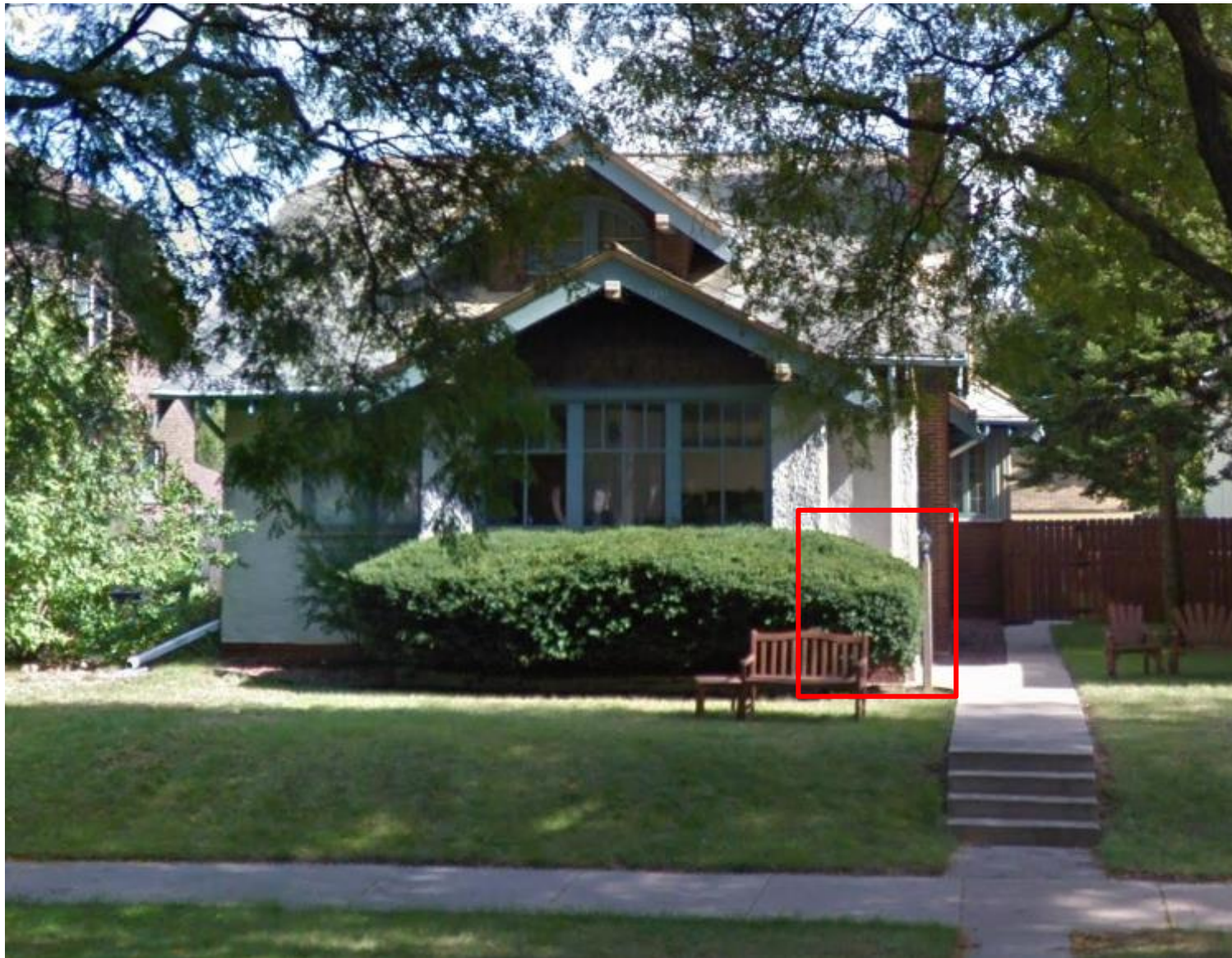
(West Elevation) Photograph of the property facing East – location of masonry columns within red box
