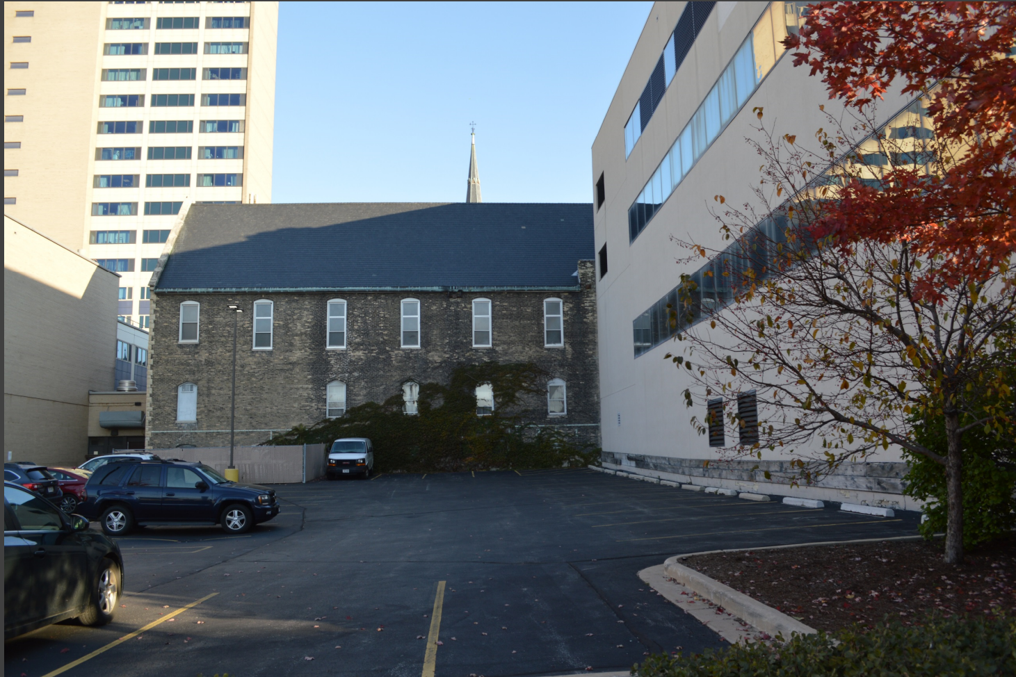
PARISH HOUSE SOUTH FACADE
