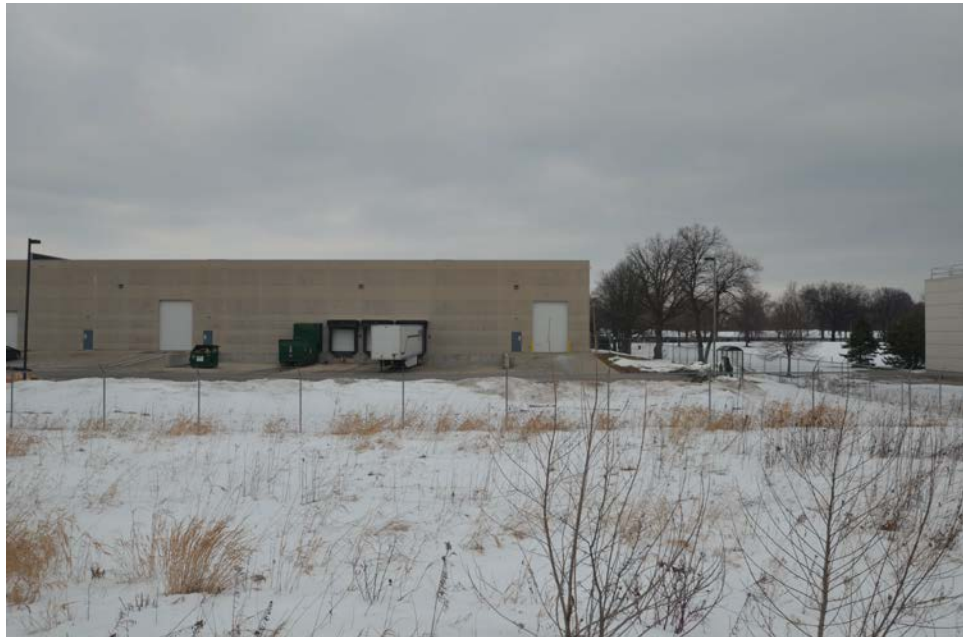
Looking North – View of existing facility at location of proposed addition
