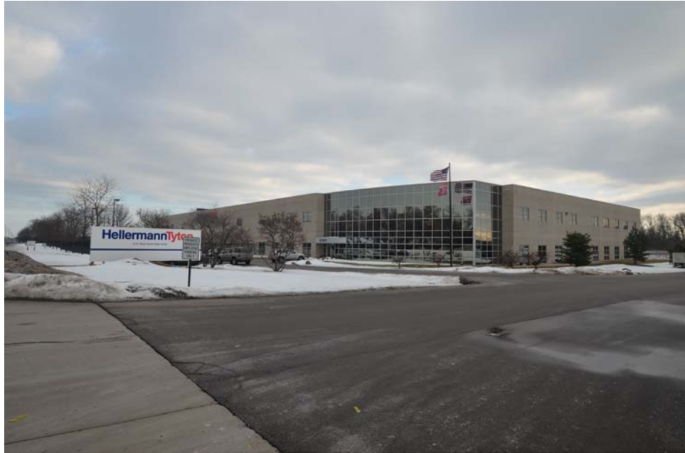
Looking Southeast – View of north and west façades of existing facility.
