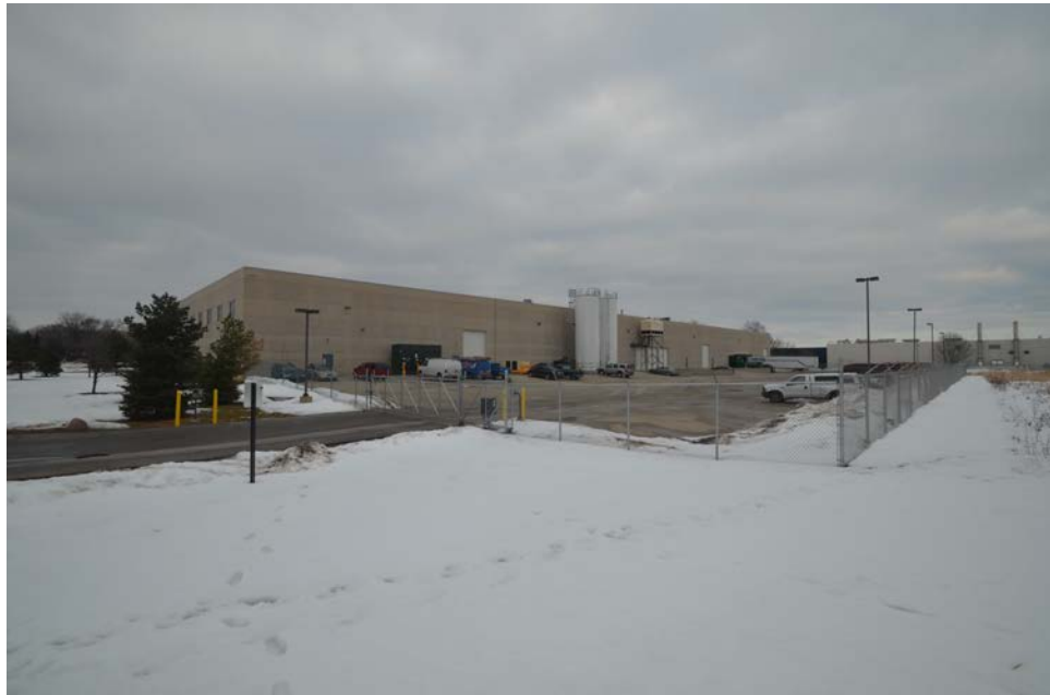
Looking Northeast – View of south façade existing facility.
