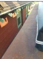
• The rubber roof adjacent to the steel cap is leaking due to poor installation.
