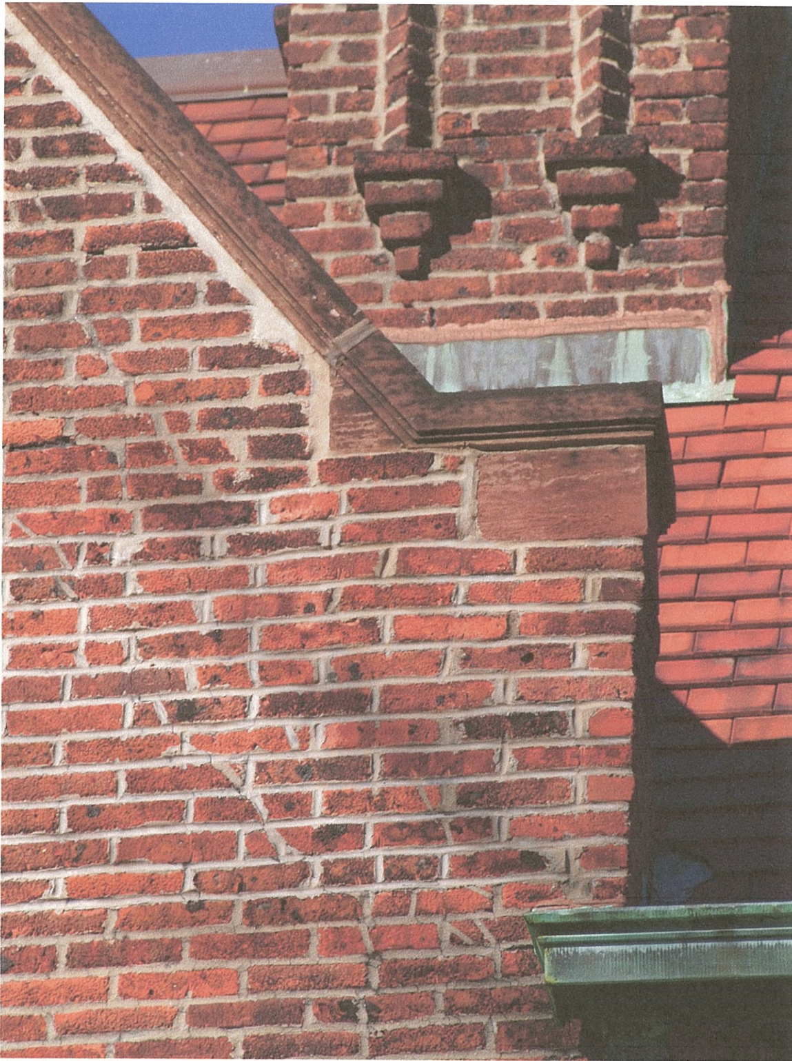
Cracked gable parapet walls – East Elevation, Charles Allis House. Condition is typical of all gables but to varying degrees. Note repaired cracks have re-cracked. Note condition of chimney in background.
