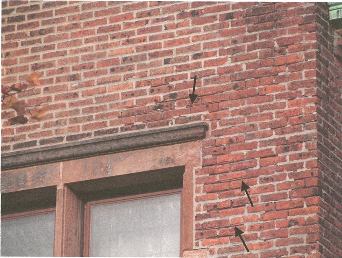
SE Corner – Charles Allis House. Wind blown runoff has repeatedly deteriorated the masonry in this area. Note the overcut bricks from a previous repointing project.
