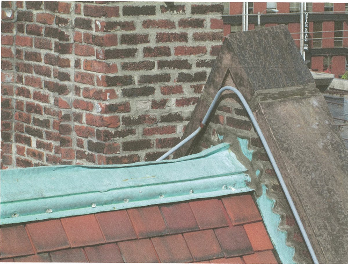
Crushed & Loose Ridge Cap – NW corner of Charles Allis House. Note excessive use of sealant on flashing, brick, and coping.
