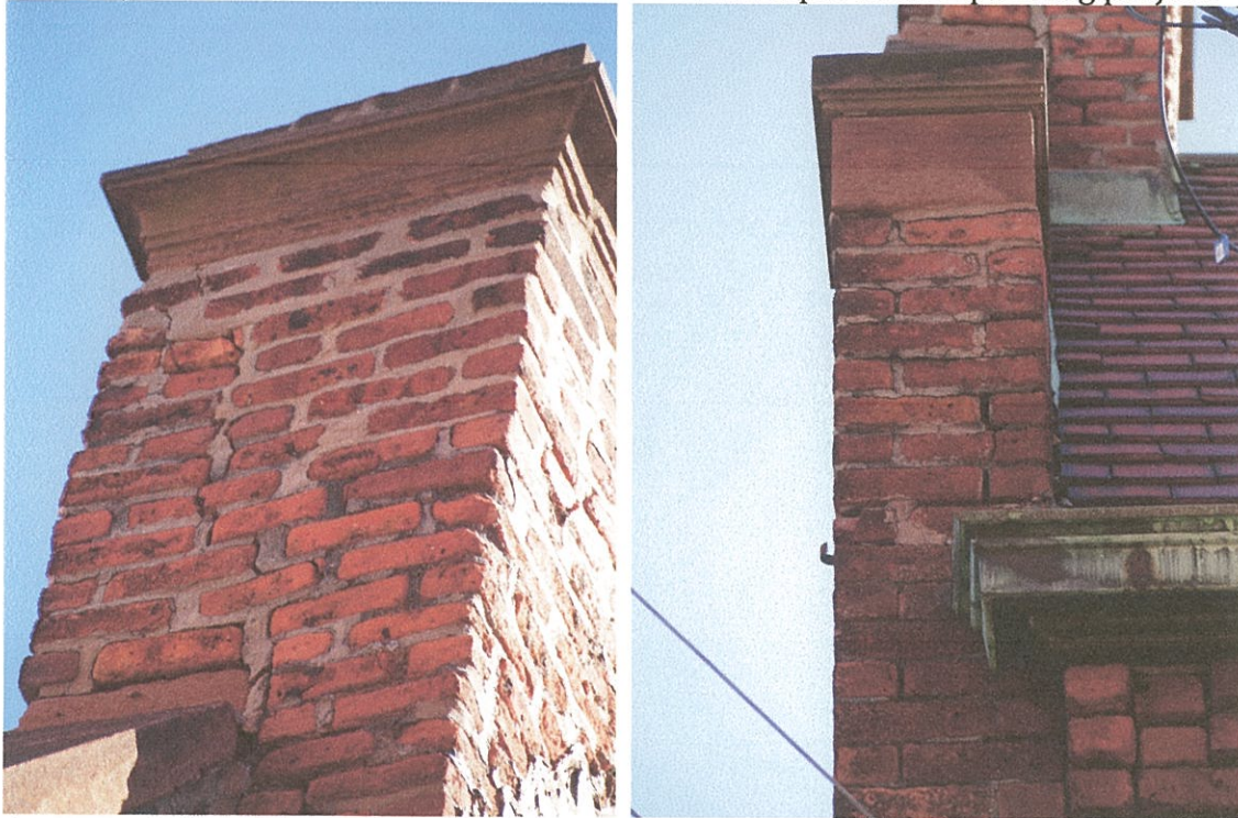
Garage North Gable & Chimney Deterioration – Charles Allis House. The leaning of the gable and chimney, along with the cracks, brick displacement required reconstruction of these elements.
