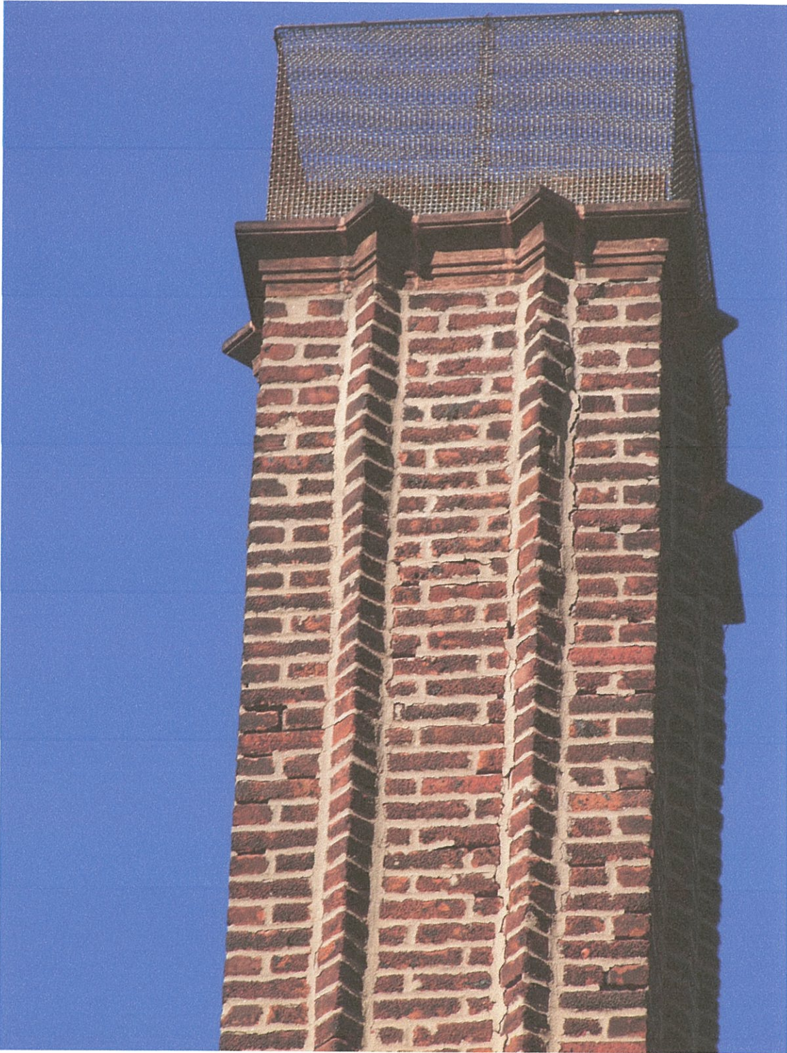
Typical Chimney Condition – East Chimney, East Elevation – Charles Allis House. Excessive spalling of hard grey pointing mortar and join cracking with brick displacement of stacked rotated brick accents.
