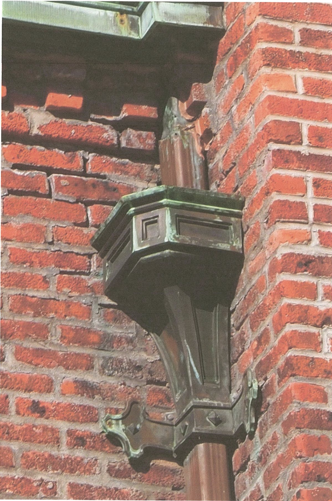
Mortar Deterioration at Downspouts, South Elevation – Charles Allis House. Typical at all downspouts.
