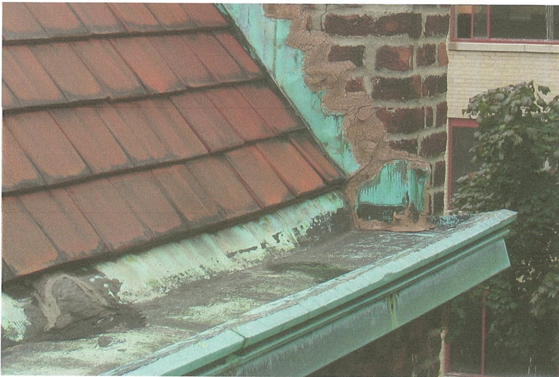
1.5" Deep Gutter at Termination - East Elevation, Charles Allis House
