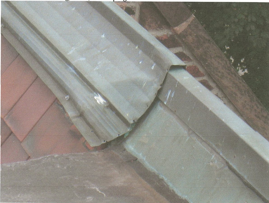
Loose Ridge Cap – NE Corner of Charles Allis House. A previous replacement, this cap was subsequently peeled open by wind or roof tile repair.
