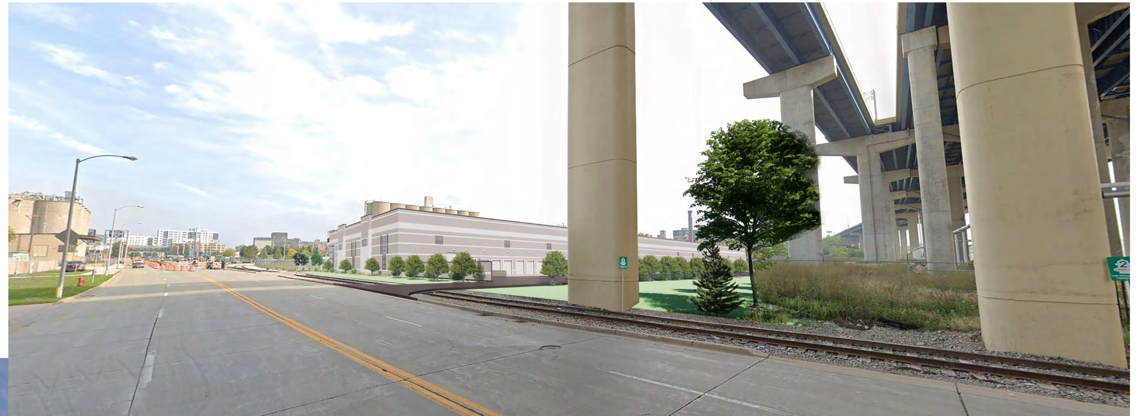
VIEW FROM NORTHWEST LOOKING EAST
