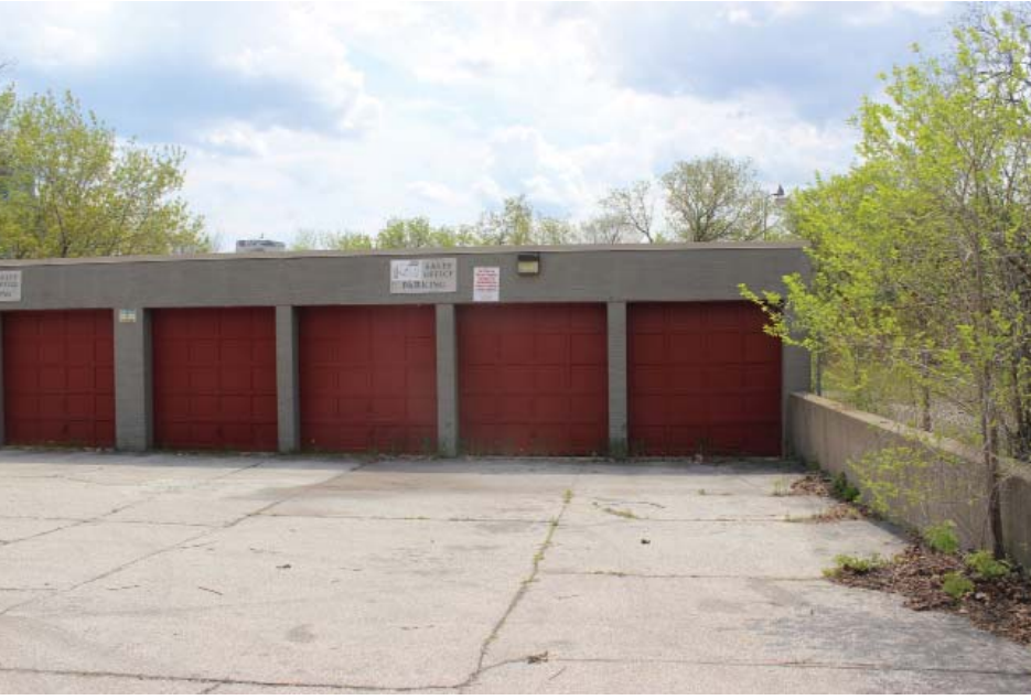
Block A existing structure
