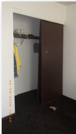
FIGURE 1 DESCRIBED AS "CLOSET DOORS OFF HARDWARE TRACK"
