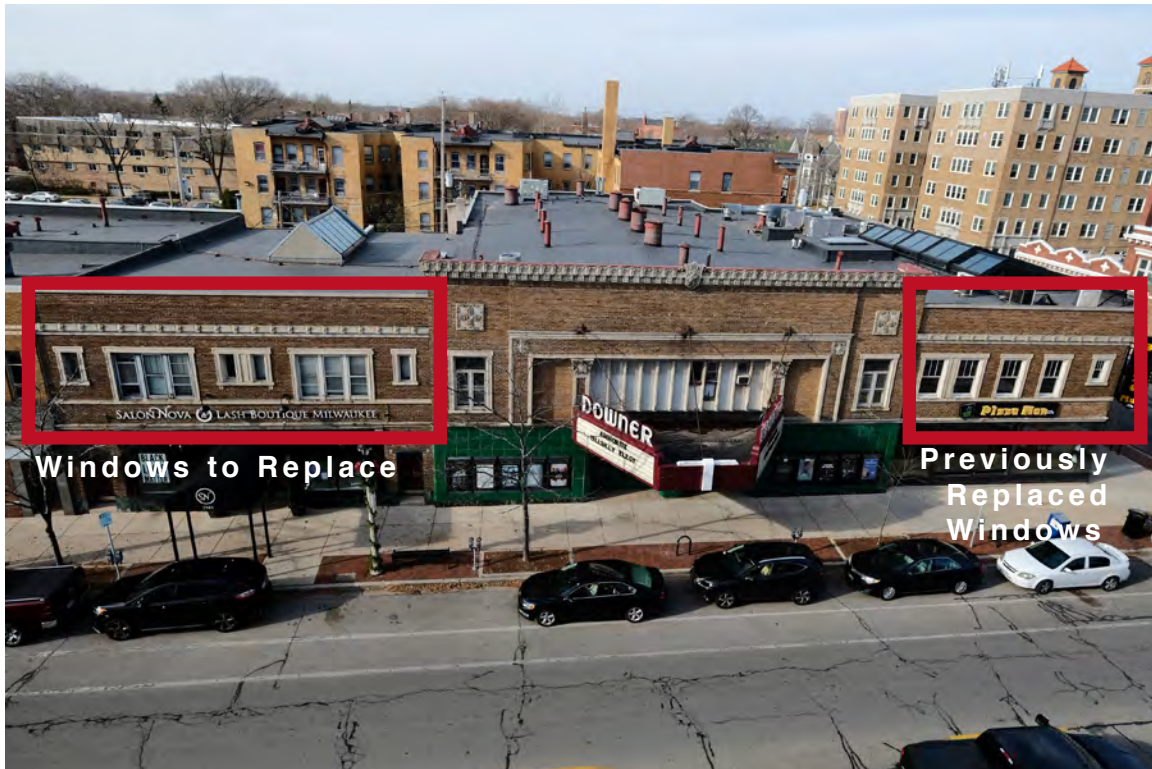
IMAGE 31: View of the Downer Theater building from across North Downer Avenue. The new windows on the south apartments will match the existing units in configuration. Preserve, LLC 2021.
