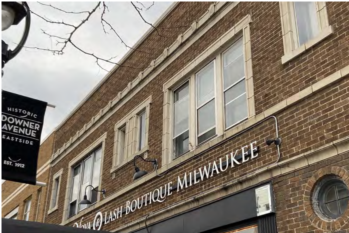
IMAGE 32: View of windows to be replaced on the second floor of the Downer Theater. Preserve, LLC 2021.
