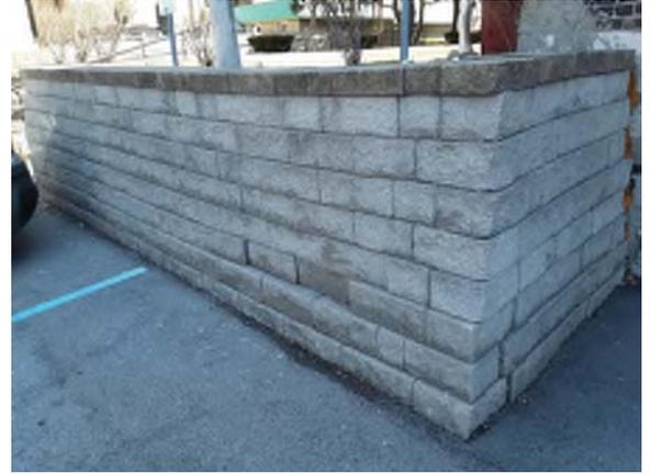
Example of Similar Replacement Material Split-Face Masonry Units Presently Used at Retaining Wall on South End of Parking Lot
