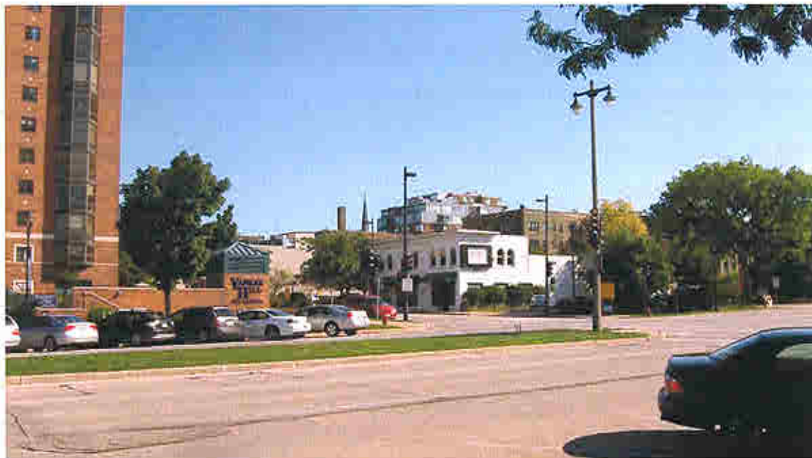
4 - VIEW OF SUBJECT PROPERTY NEAR INTERSECTION OF KILBOURN & VAN BUREN
