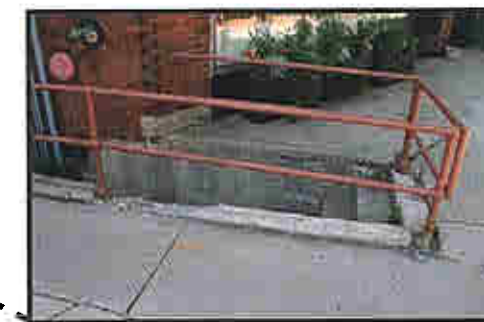
STAIR AND RAILING
