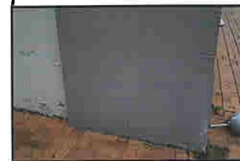
CONCRETE PIER COVER
