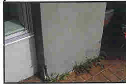
CONCRETE PIER COVER
